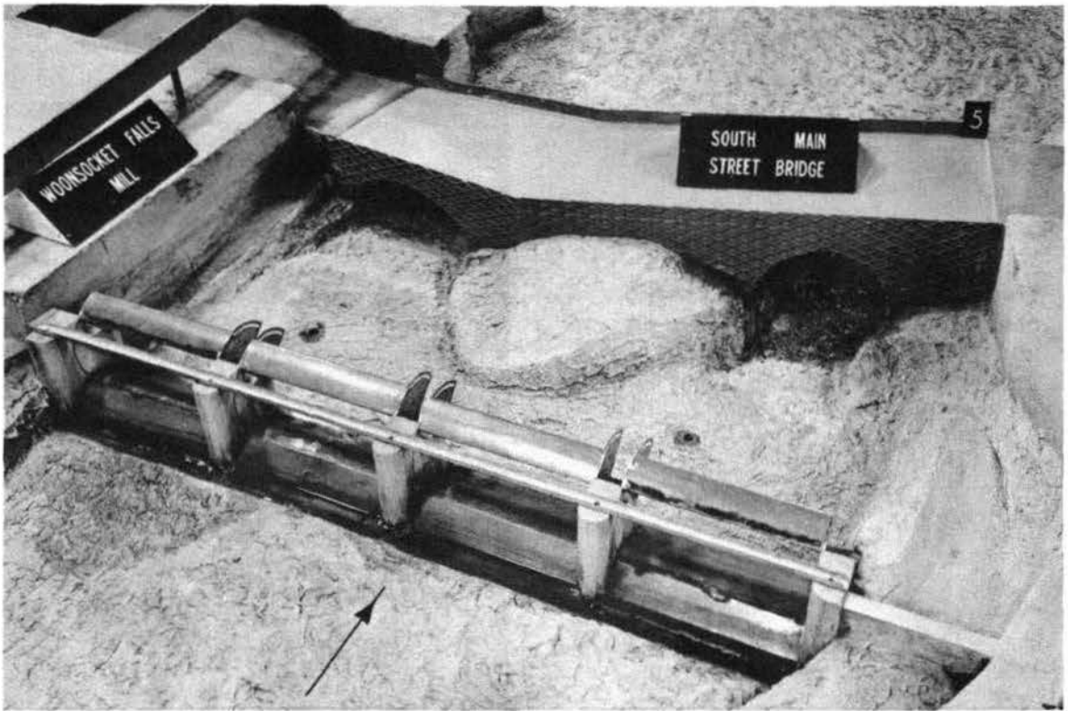
Photograph 3. Original design: Woonsocket Falls Dam and rock excavation between dam and South Main Street bridge
