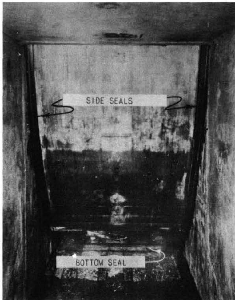
Fig. 4. Upstream face of gate
