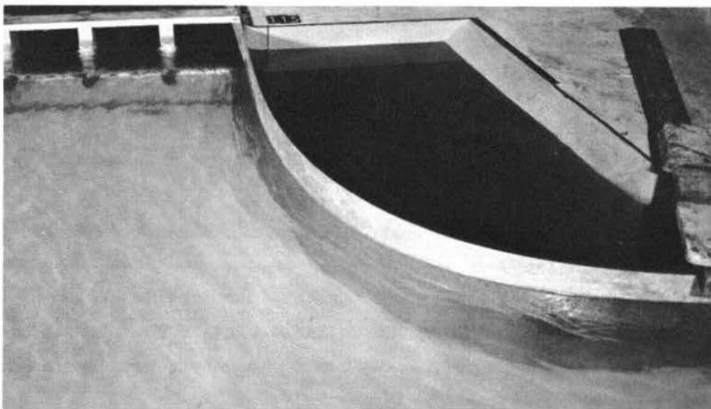
Fig. 5. Flow at right abutment Discharge, 586,000 cfs; pool elevation, 1221.6
