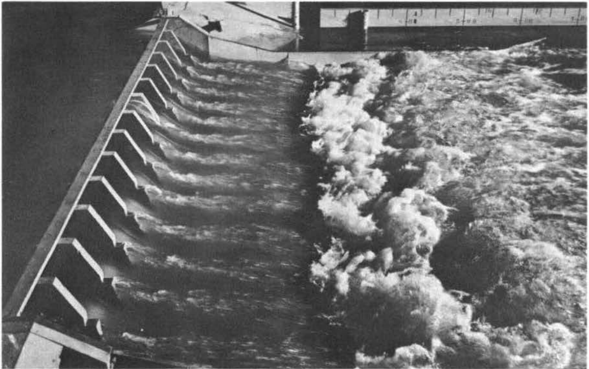
Fig. 6. Height of chute walls was adequate for maximum flow in chute. Discharge, 626,000 cfs; pool elevation, 1223.5; and tailwater elevation, 1176.3
