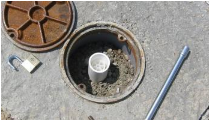
Multilevel Well Construction
