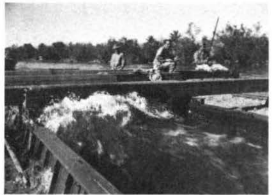
Two-ponton M4 raft -- normal spacing Pontons with 10-in. freeboard in still water being towed about 8 fps
