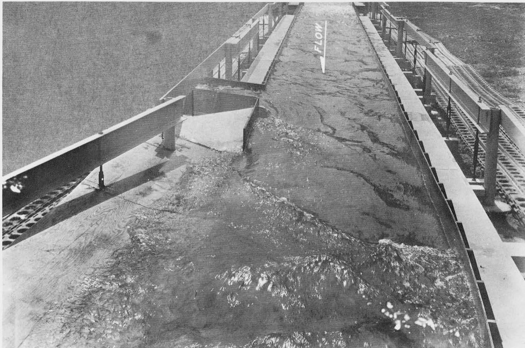
Original design, junction Tophet Brook Discharge: Hoosic River 8,200 cfs; Tophet Brook 2,000 cfs
