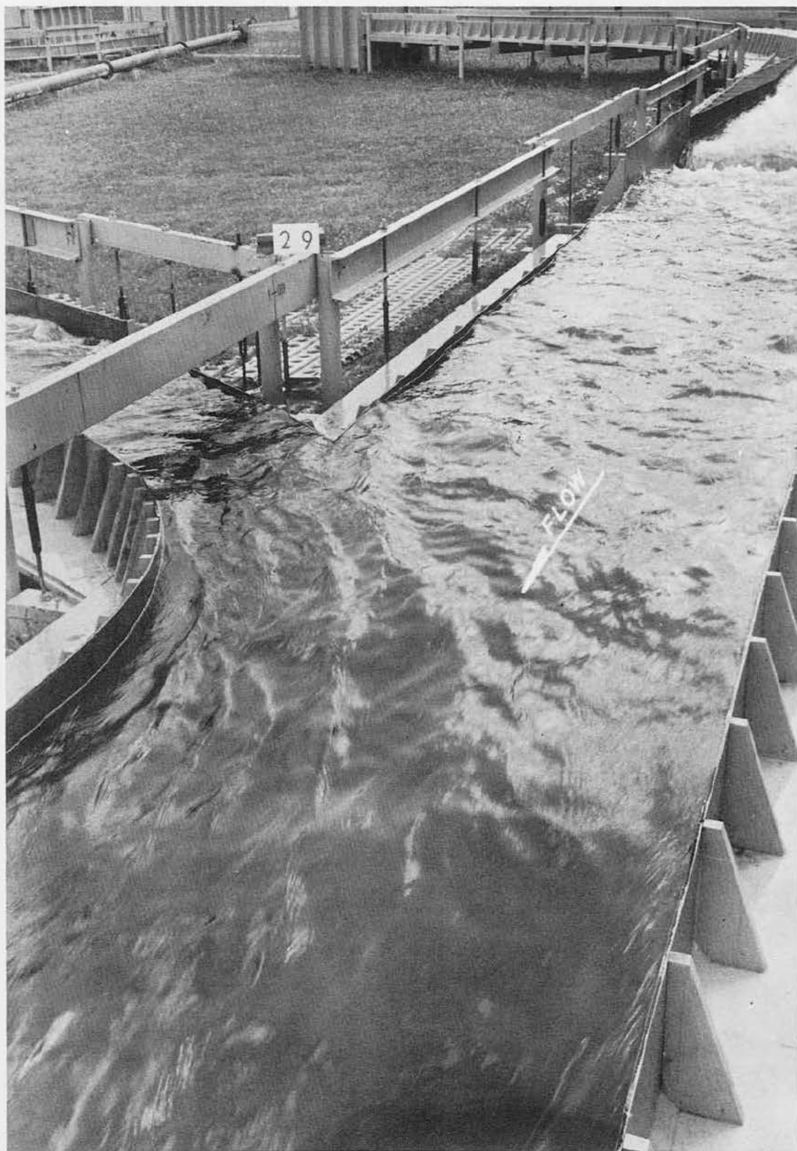
Plan 4, revised junction of Tophet Brook with Plan 3 channel Discharge: Tophet Brook 2,000 cfs; Hoosic River 13,000 cfs
