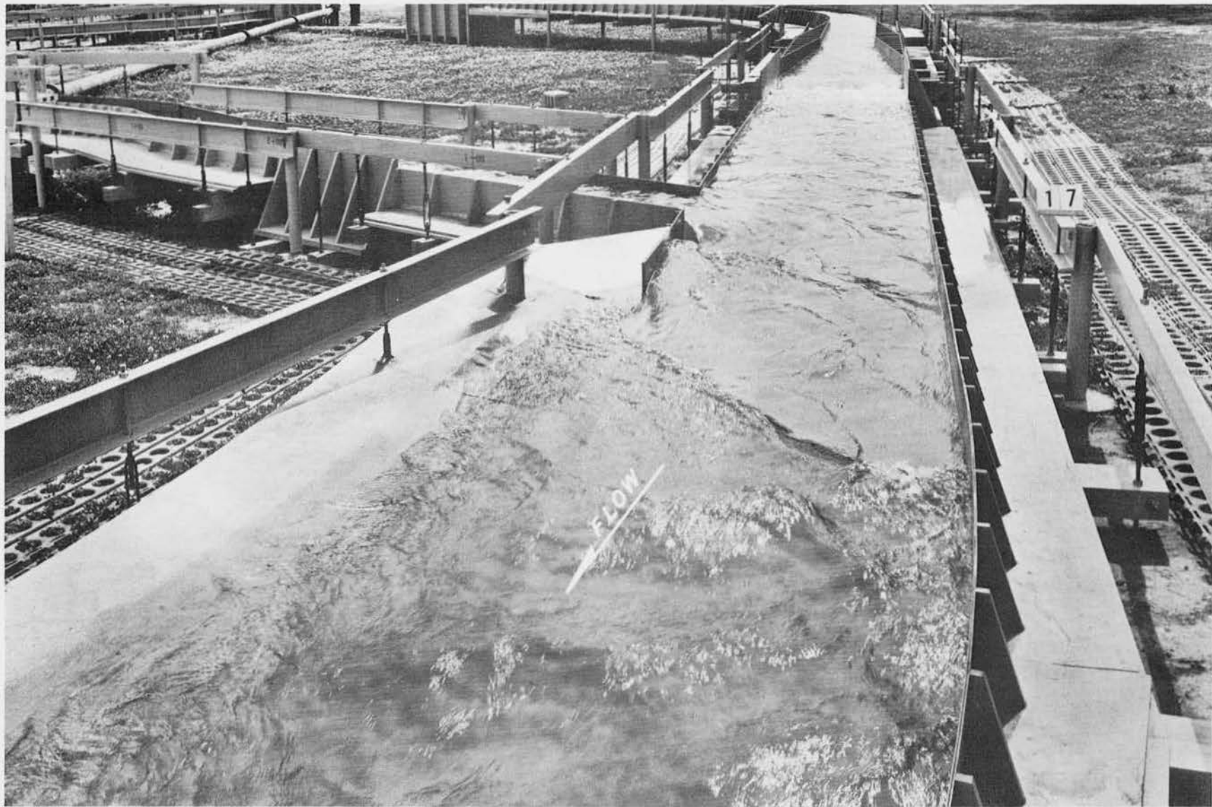
Original design, junction of Tophet Brook with Plan 3 channel Discharge: Tophet Brook 2,000 cfs; Hoosic River 8,200 cfs
