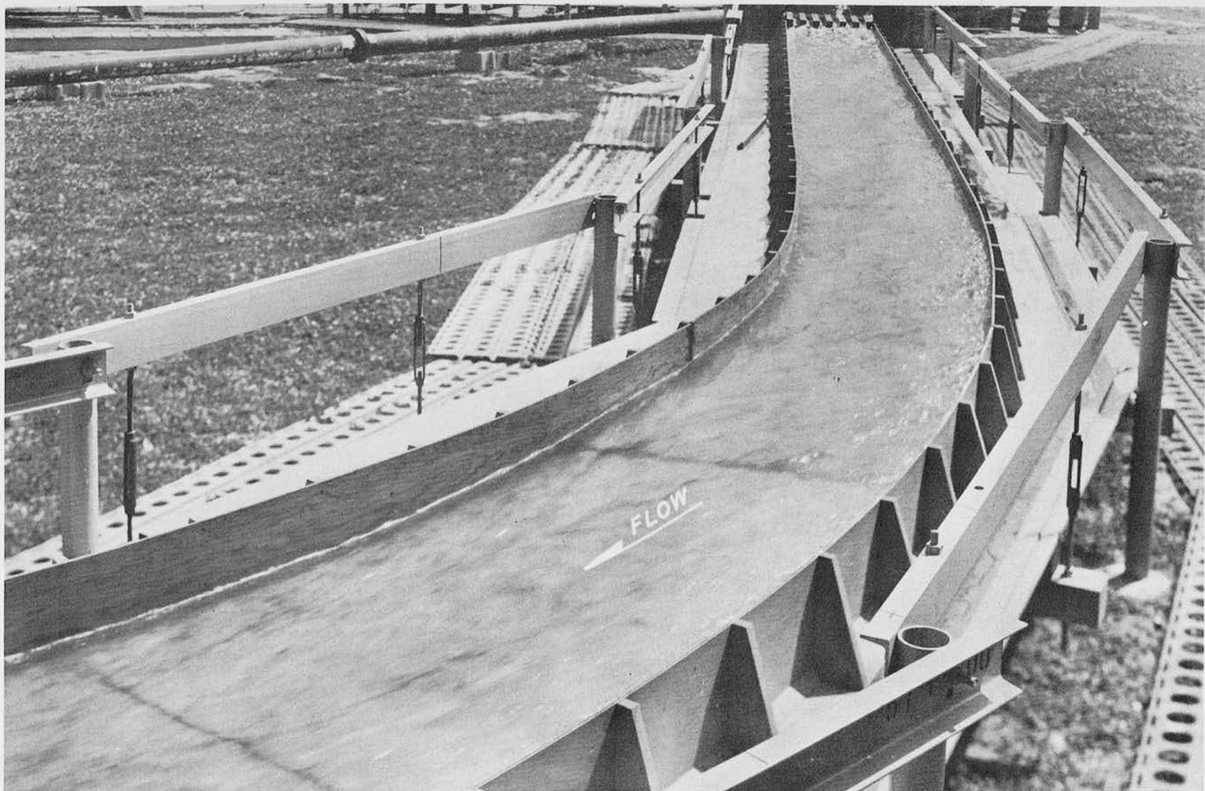
Original design, main channel. Station 63+00 to station 55+00 Discharge 13,000 cfs
