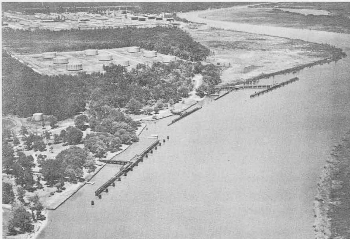
Fig. 2. Vincent Landing on Calcasieu River about 6 miles south of Lake Charles. A sulphur tank farm is in foreground, refining company beyond.
