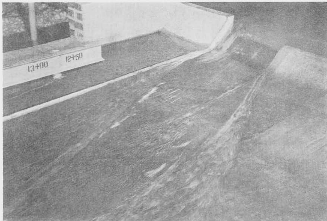
Figure 14. Exit channel flow with 100-ft low weir at right abutment; discharge 172,000 cfs, type H
