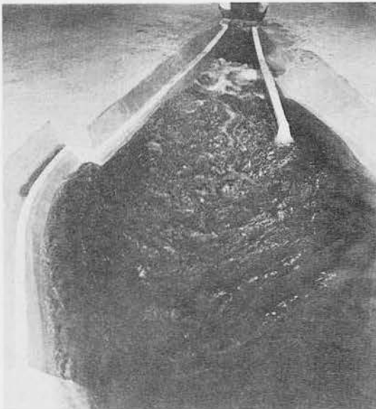
Discharge, 3,500 cfs; tailwater, 1529.5
