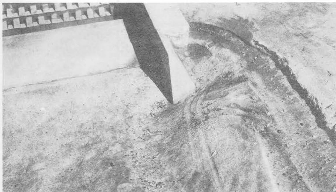
Upstream view showing scour below the left training wall after 1 hr of operation
