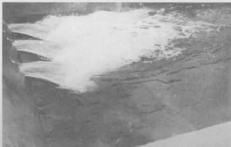
b. All sluices in operation Discharge 16,950 cfs Tailwater elev 496.7
