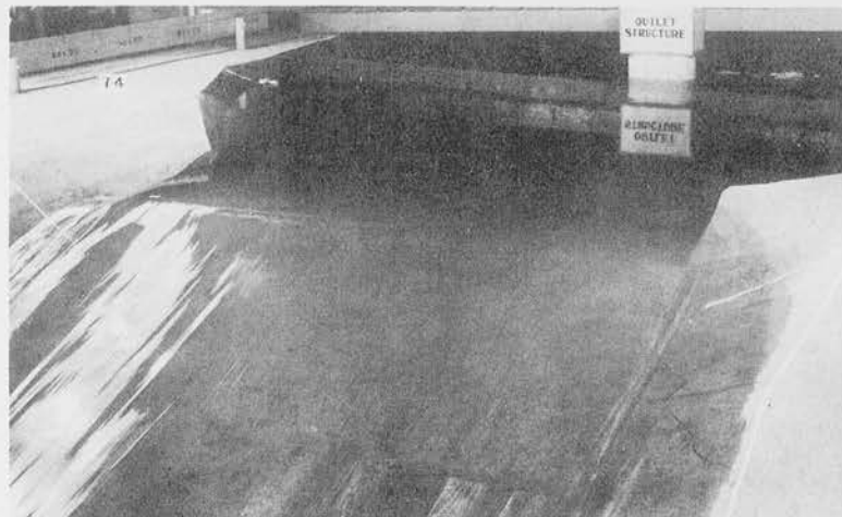
Type A walls. Discharge 25,000 cfs
