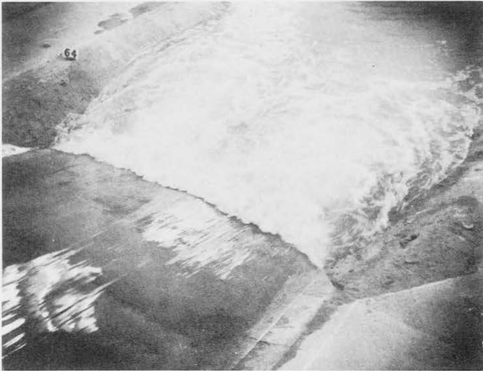
Discharge 25,000 cfs; tailwater elevation 216.0
