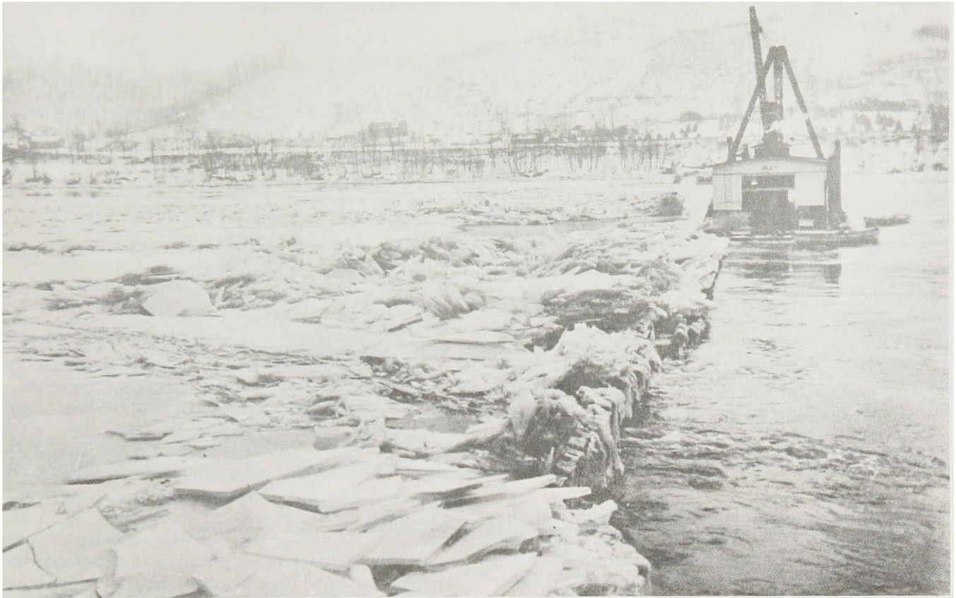
A wicket dam on the Ohio River on 28 December 1935. Maneuverboats normally carried on their operations on the upstream side of the dam. Here, ice conditions made it necessary to work from the downriver side
