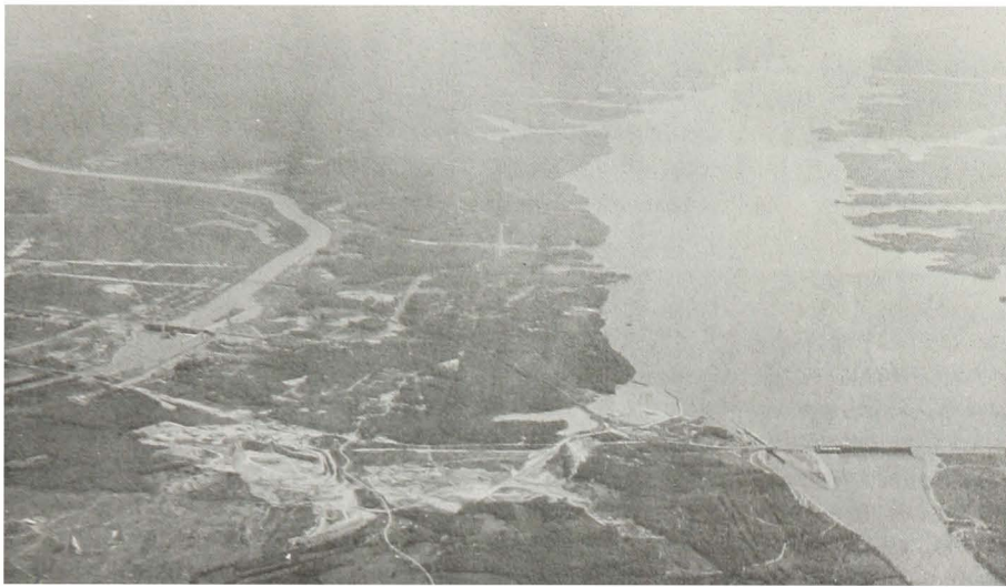
Barkley Lock and Dam under construction on Cumberland River (left) in 1963. Barkley Canal is being excavated in the dry to connect with Kentucky Lake (right)
