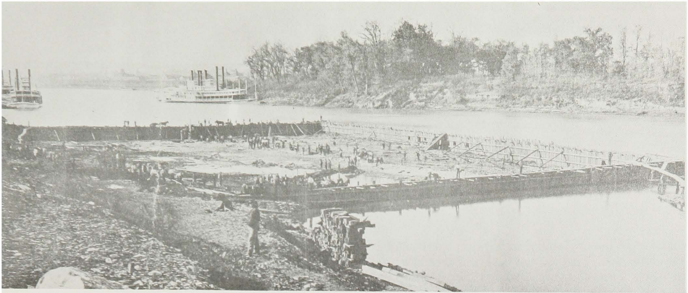
Rebuilding of the Louisville and Portland Canal, 1873. Photograph from Record Group 77 of National Archives
