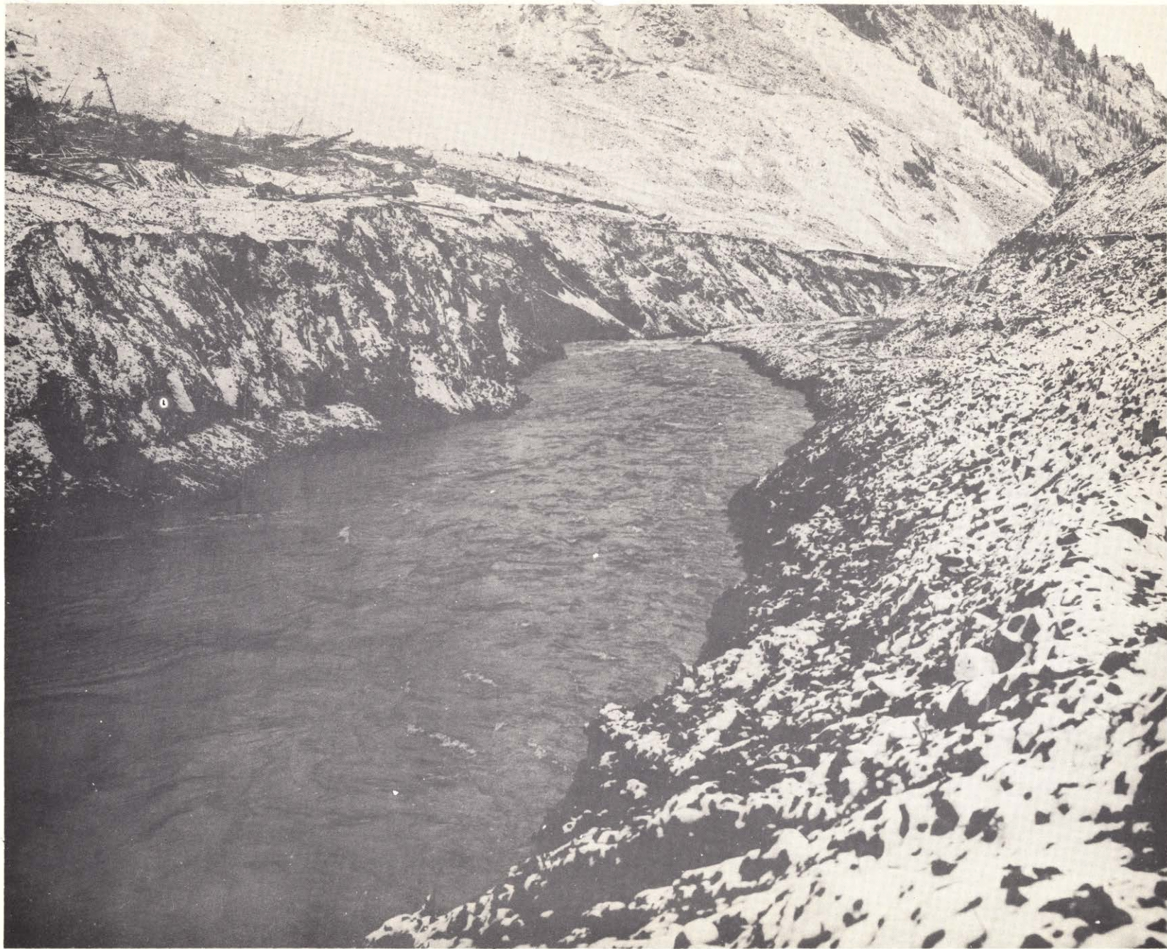
Photo 26. 29 October 1959. Completed spillway looking downstream from about Station 30+00.
