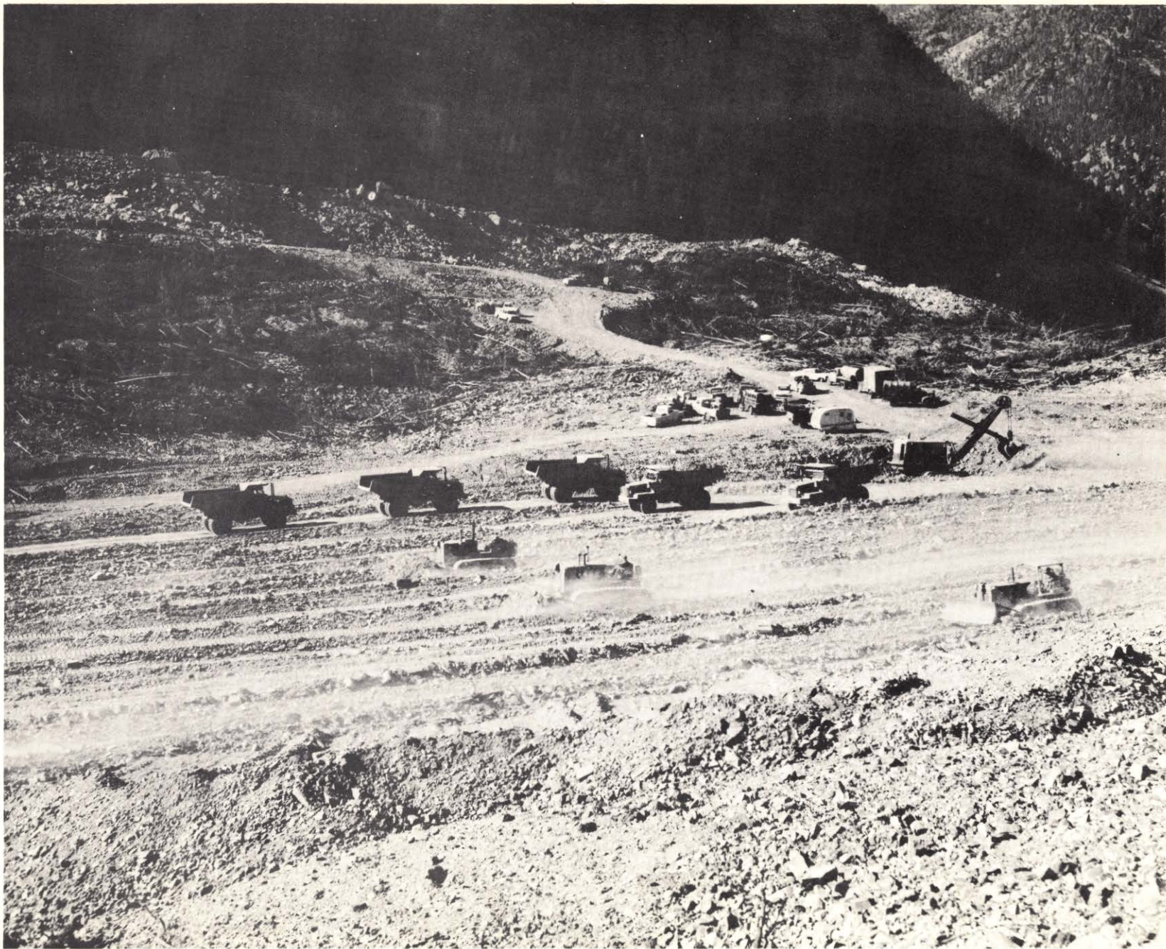
Photo 4. 28 August 1959. Equipment constructing initial spillway.
