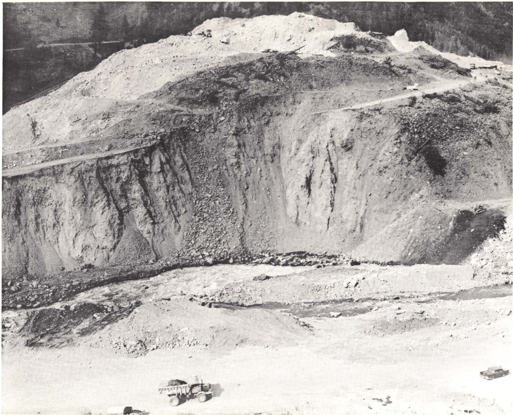
Photo 17. 5 October 1959. Rapid erosion of right bank between Stations 11+00 and 15+00.
