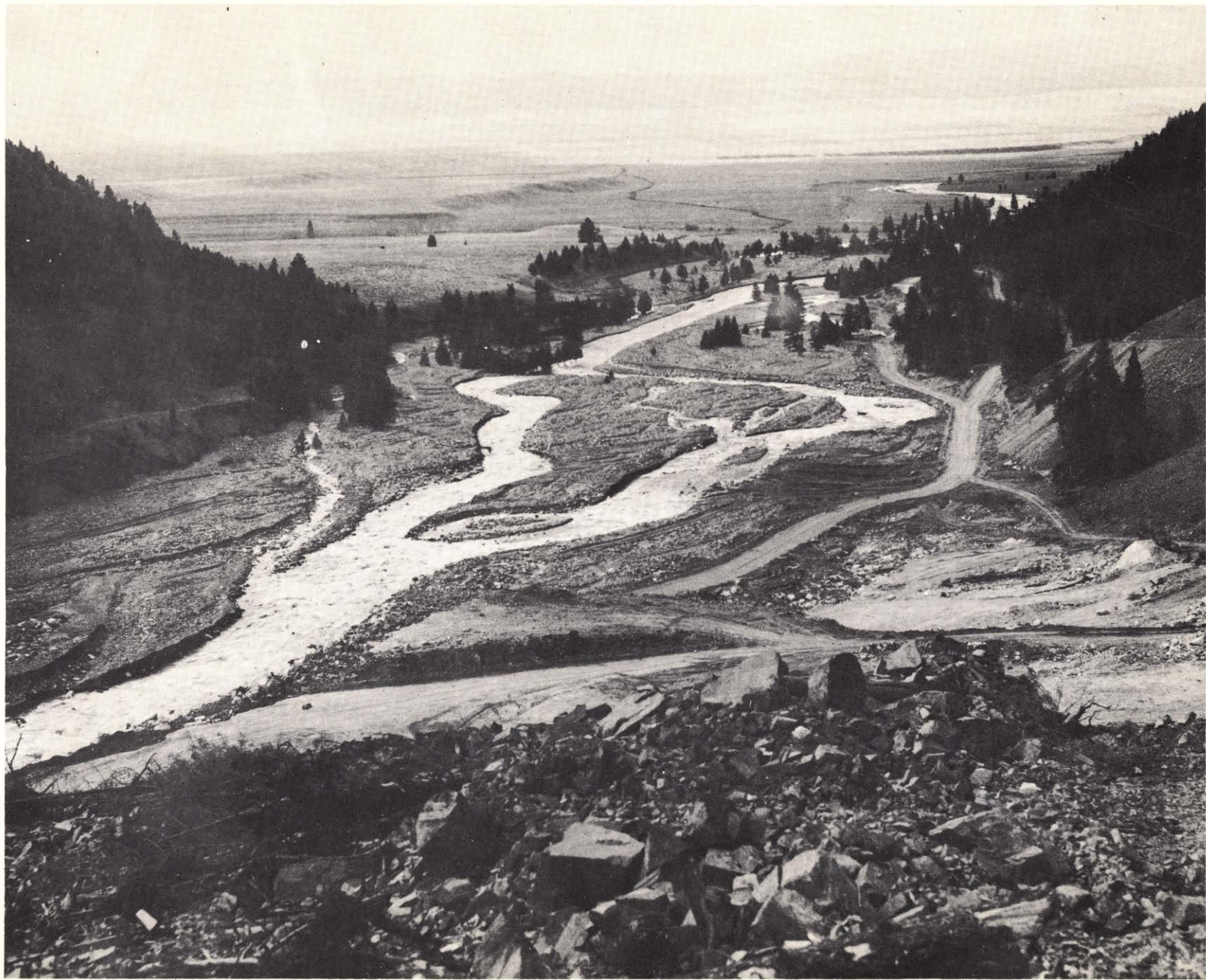
Photo 27. 28 October 1959. View of fan at lower end of slide at end of construction period (for earlier view, see Photo 2).
