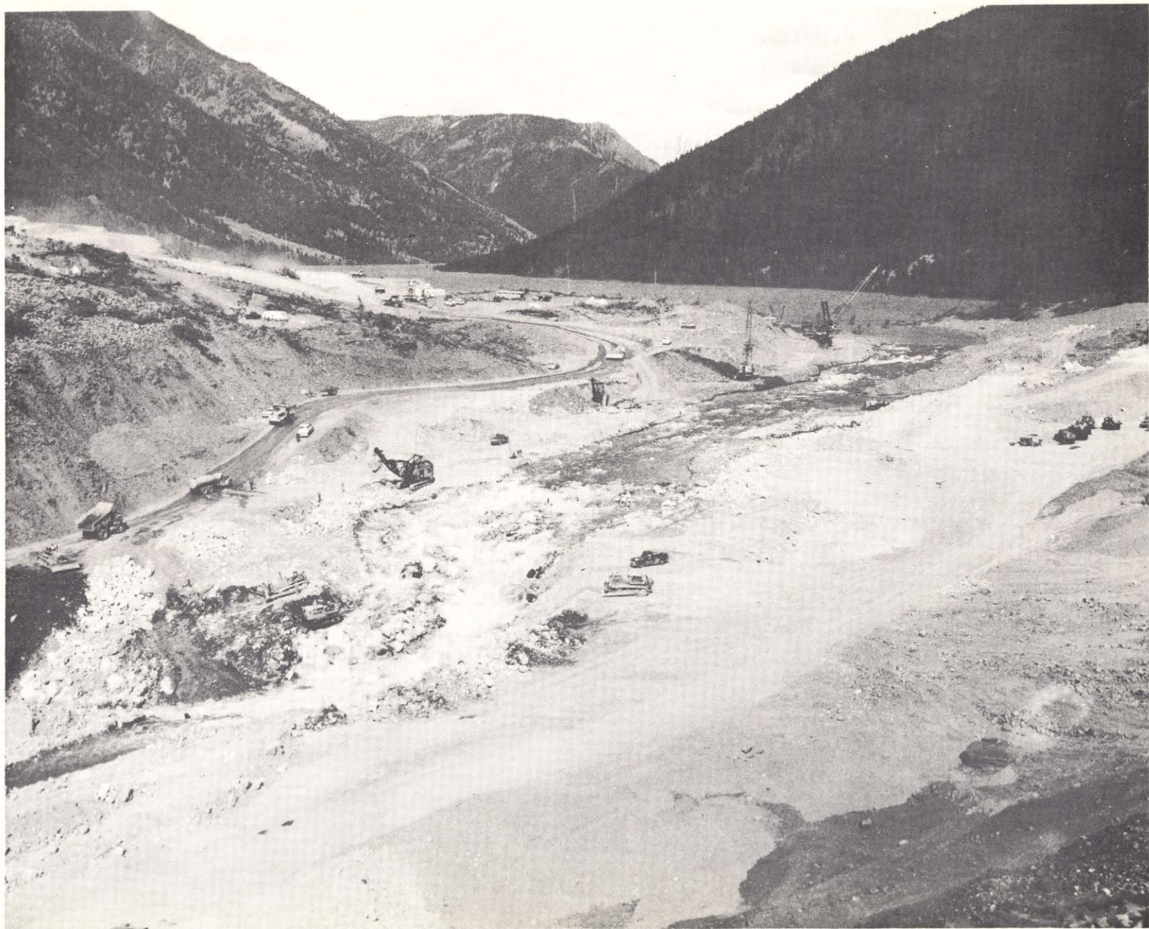
Photo 16. 5 October 1959. General view of spillway lowering operation. Draglines are working in channel and shovels are maintaining a work berm.
