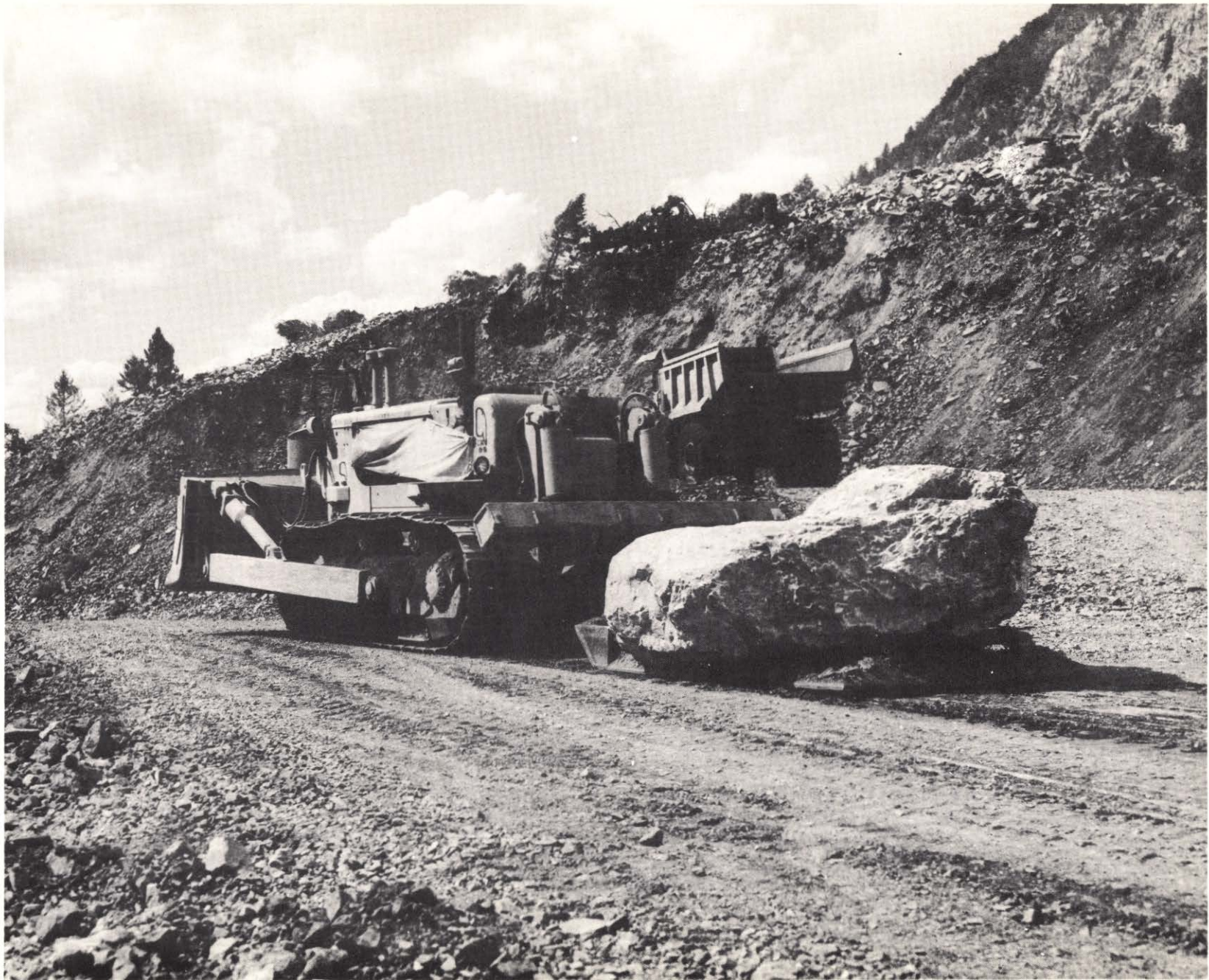
Photo 11. 16 September 1959. Tractor pulling large rock on rock sled.
