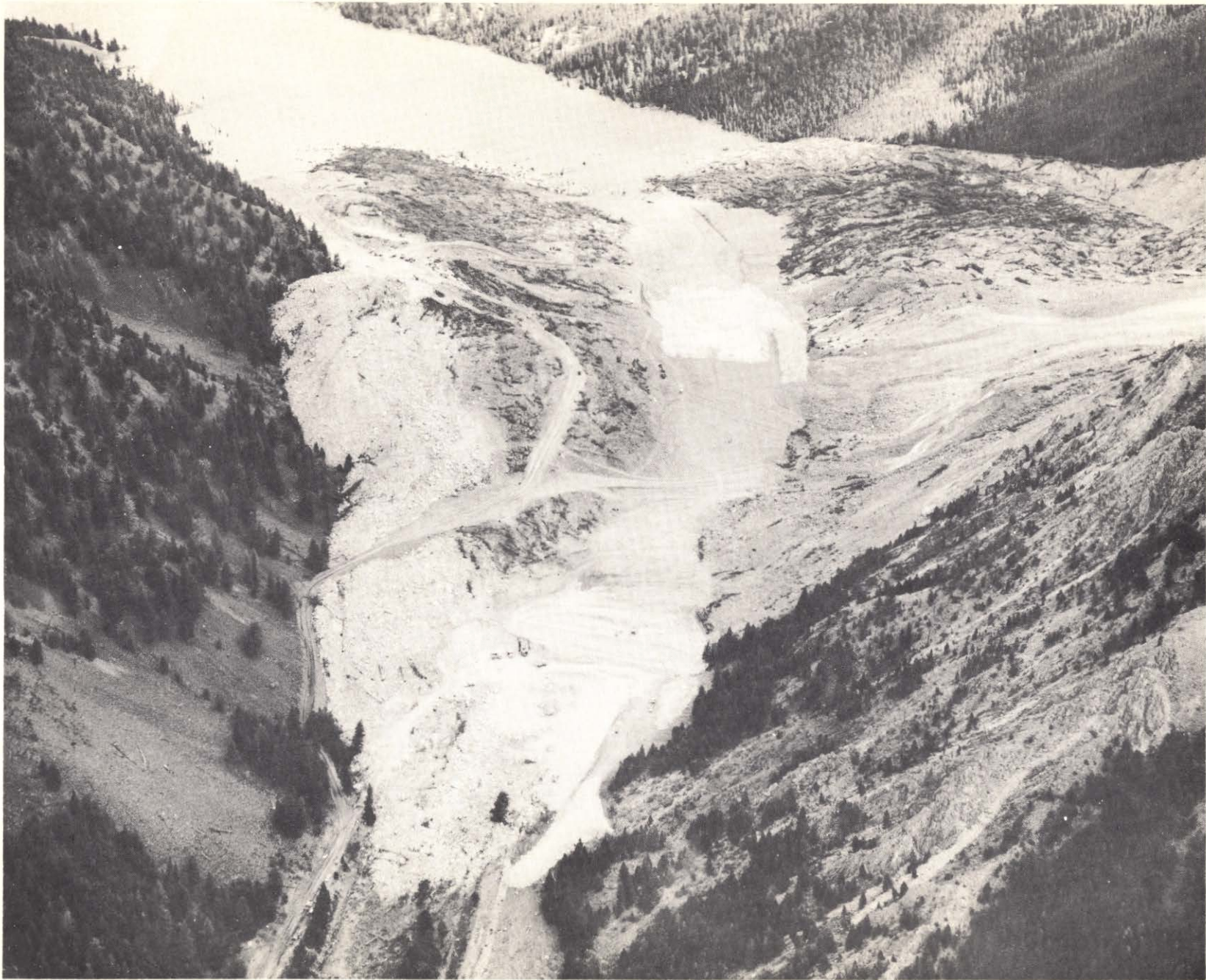
Photo 5. 3 September 1959. Aerial view of initial spillway construction.
