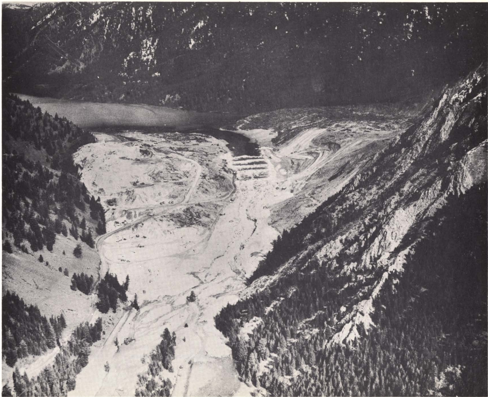
Photo 14. 22 September 1959. Aerial view of slide showing water pouring over rock terraces.
