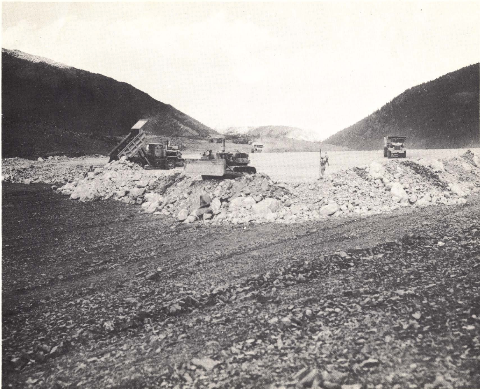
Photo 7. 4 September 1959. Placing spillway armor material in channel.
