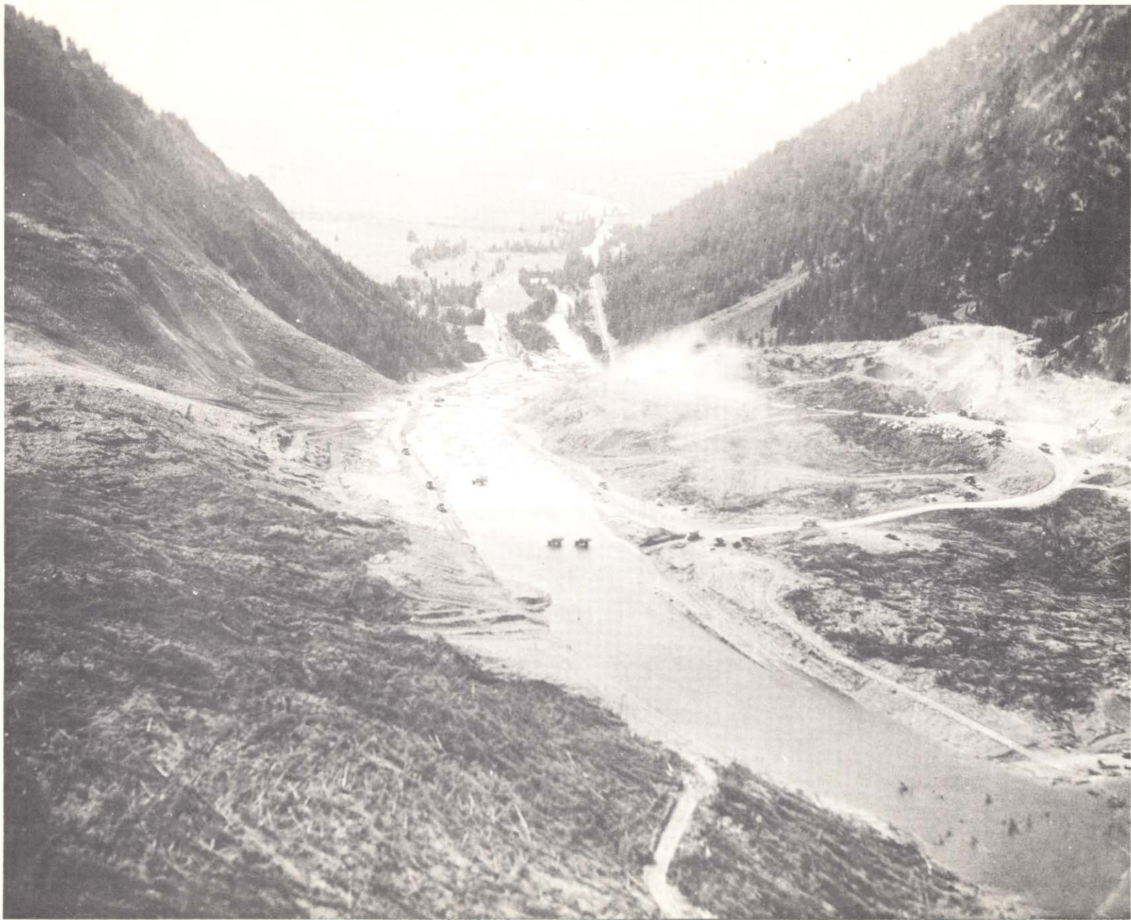
Photo 9. 11 September 1959. Downstream aerial view of water passing over slide in spillway channel.
