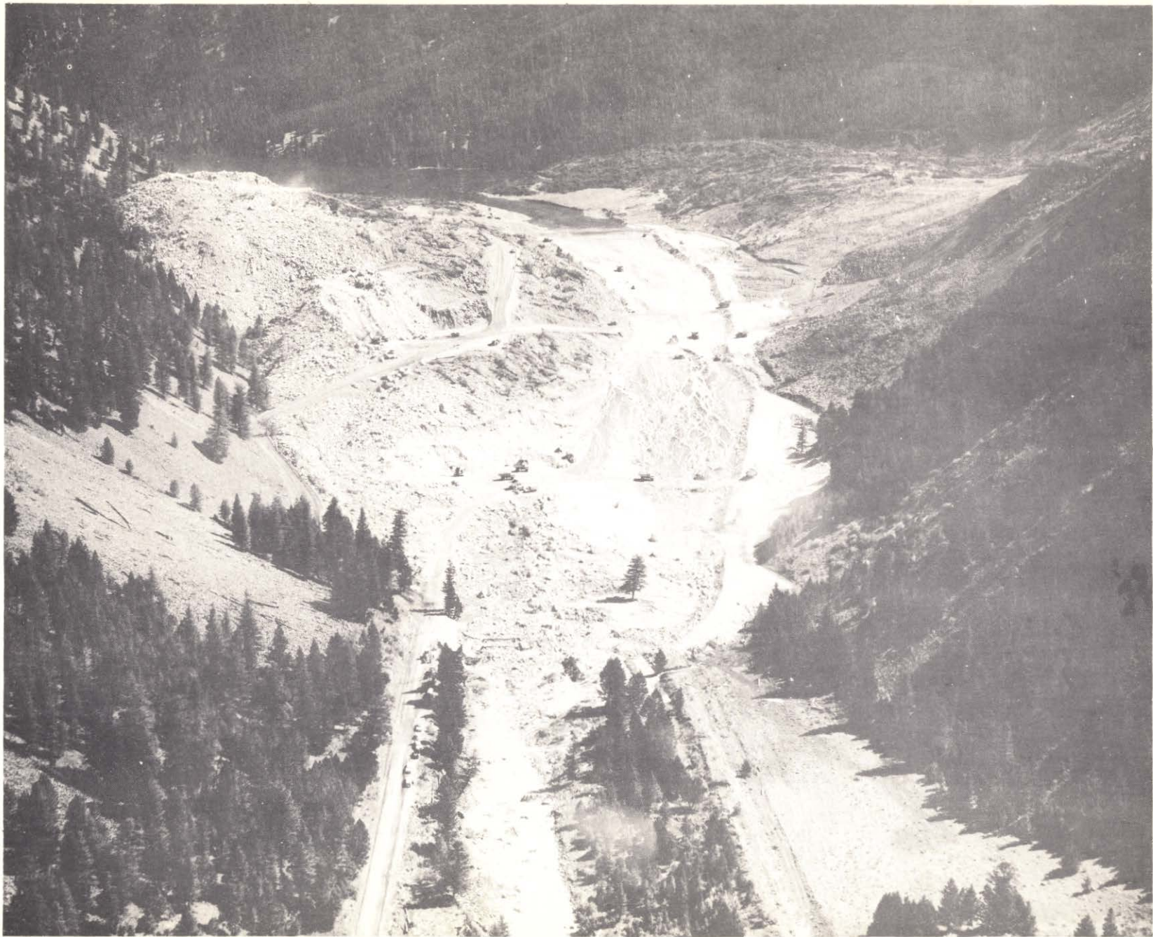
Photo 8. 10 September 1959. Upstream aerial view of spillway channel on first day water passed over slide.
