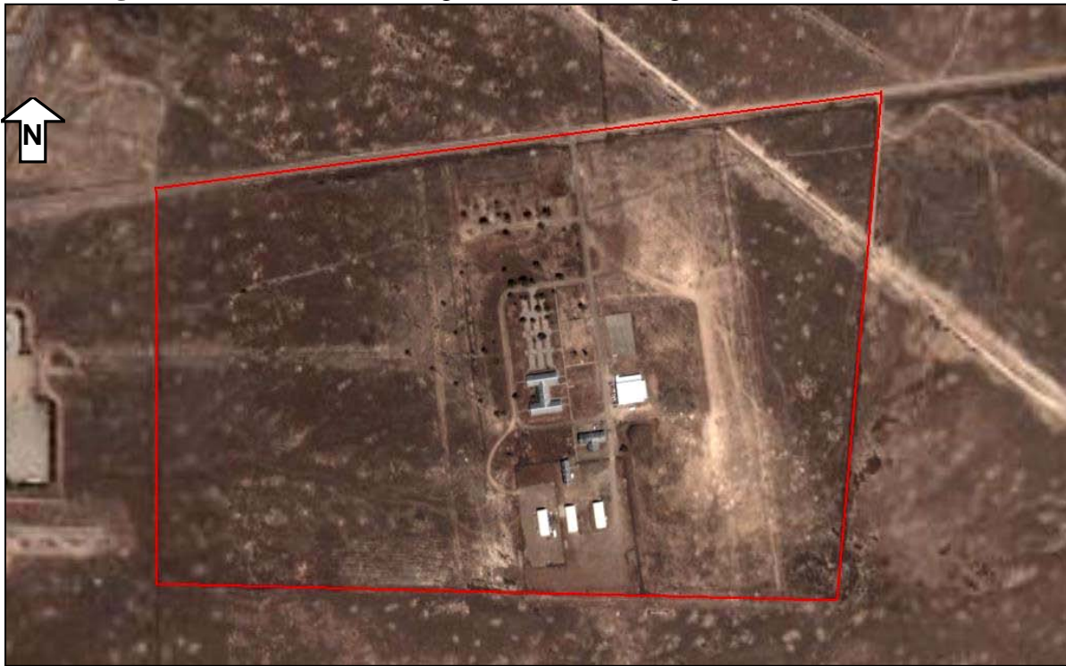
Figure 3. Overview of existing facilities at the Edgемеade Readiness Center.
