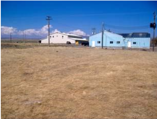
Figure 14. Areas around buildings are dominated by annual weeds and are mowed to reduce risk of fire.
