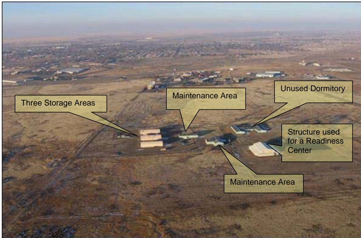
Figure 4. Photograph of existing facilities at the Edgемеade Readiness Center (facing west).
