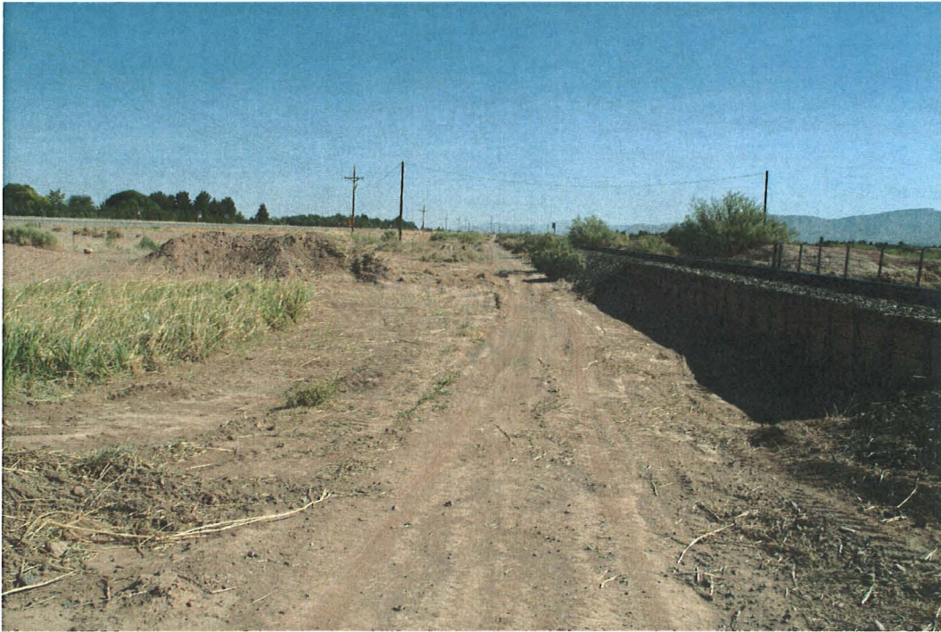
Photo 2. View of conditions at the southern terminus of the U.S. Highway 54 alternative with a typical drainage feature for the area in the foreground (10°).
