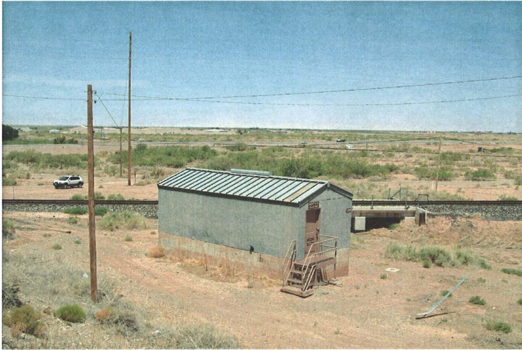
Photo 1. Photo of the pump house which serves as the common origin for all three alternative pipeline routes (Photo aspect 280°).
