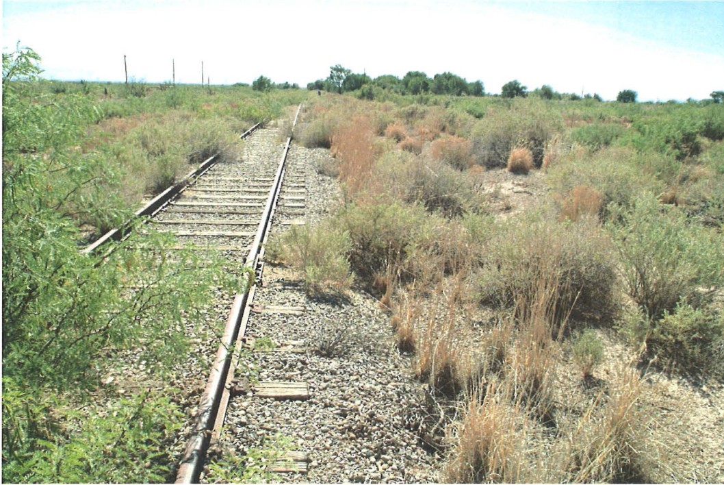
Photo 7. View of conditions along the HAFB Railroad Spur alternative (270°).
