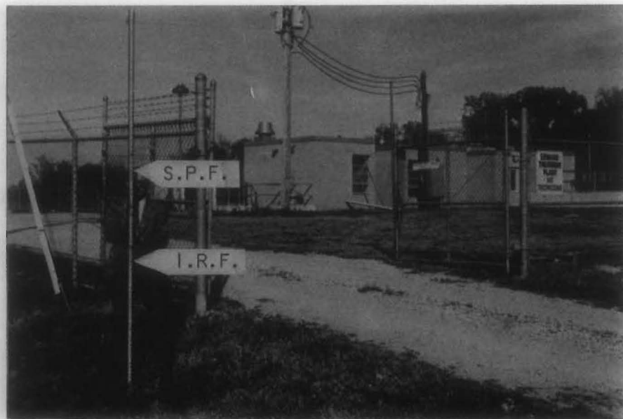
Figure 18. Depth of potential floods - Ashland Municipal Sewage Treatment Plant
