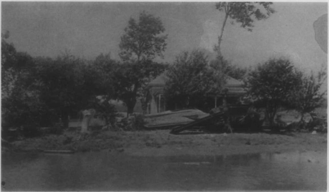
Figure 6. Flood damage on Silver Street July 1908 (Courtesy City of Ashland)
