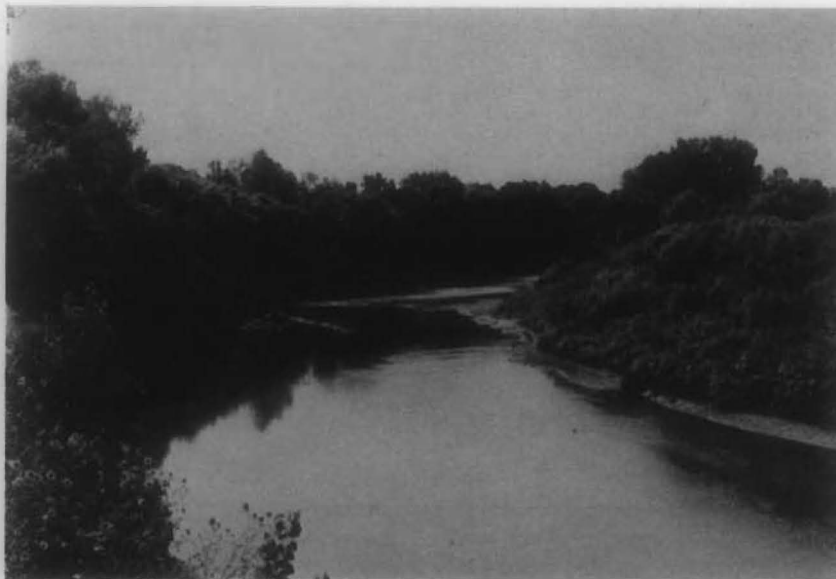
Figure 2. Salt Creek improved channel looking downstream from west line of Section 10, T12N, R9E
