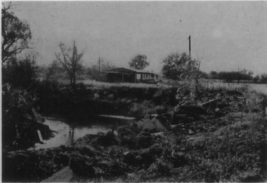
Figure 3. Development near upstream limit of Wahoo Creek
