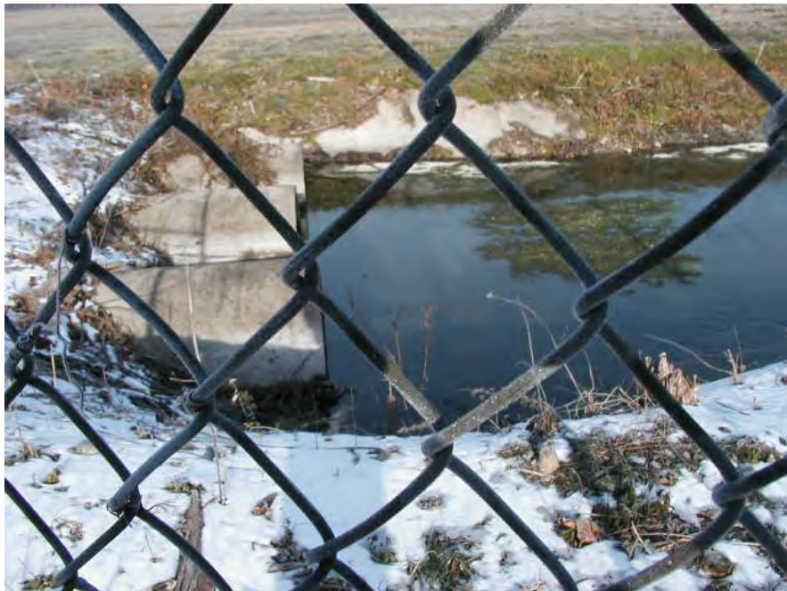
Photograph #2 – Culverts where open ditch flows beneath access road
