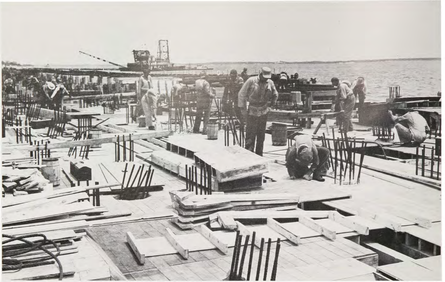
Early stage of construction at Wharf No. 2
