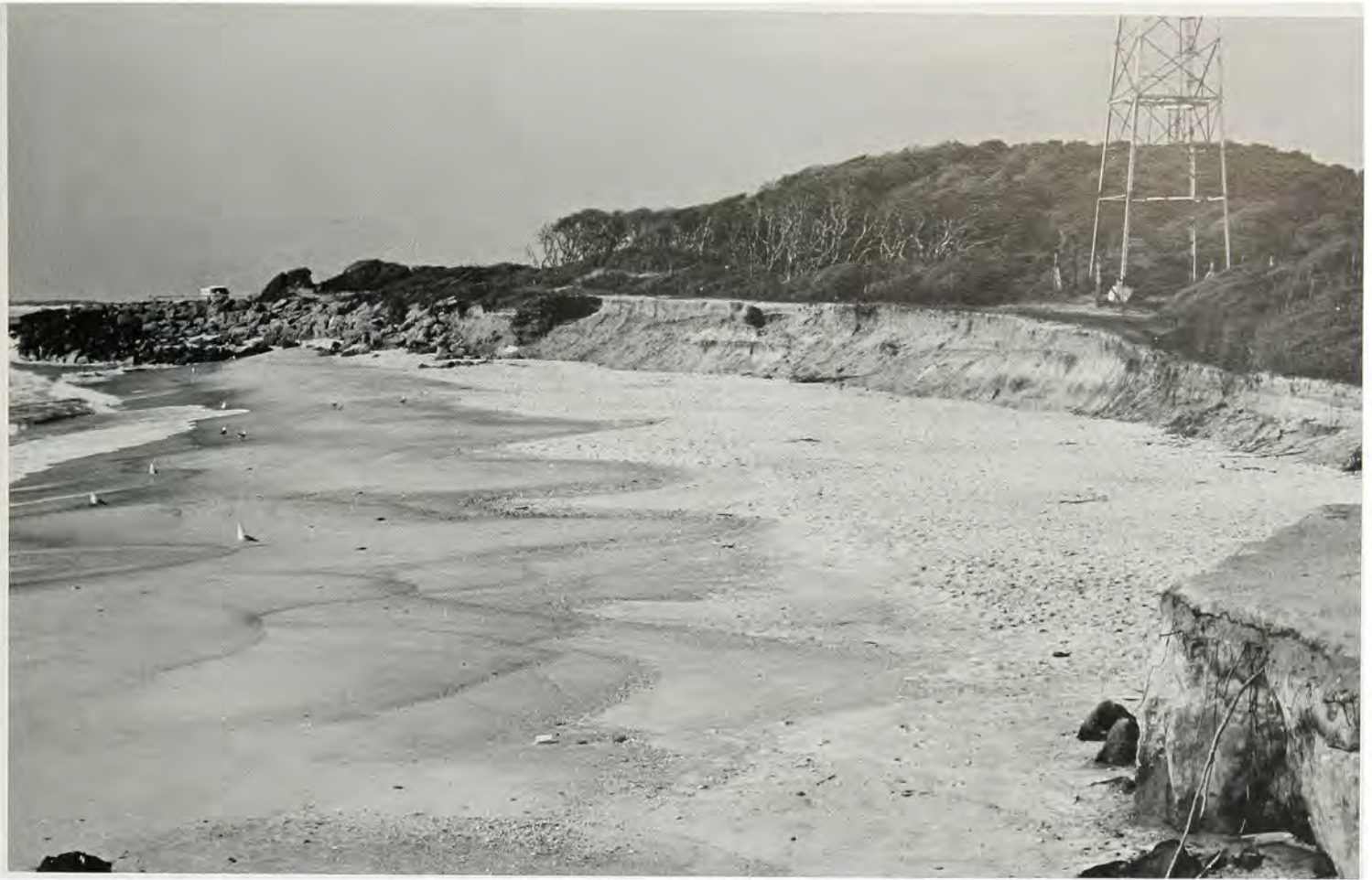
Erosion at Fort Fisher, 1982
