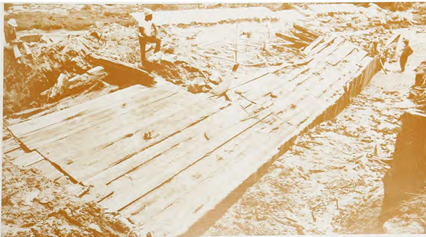
Uncovered at Falls Lake project during construction of the dam was a wooden dam built in the 1820s or 1830s.
