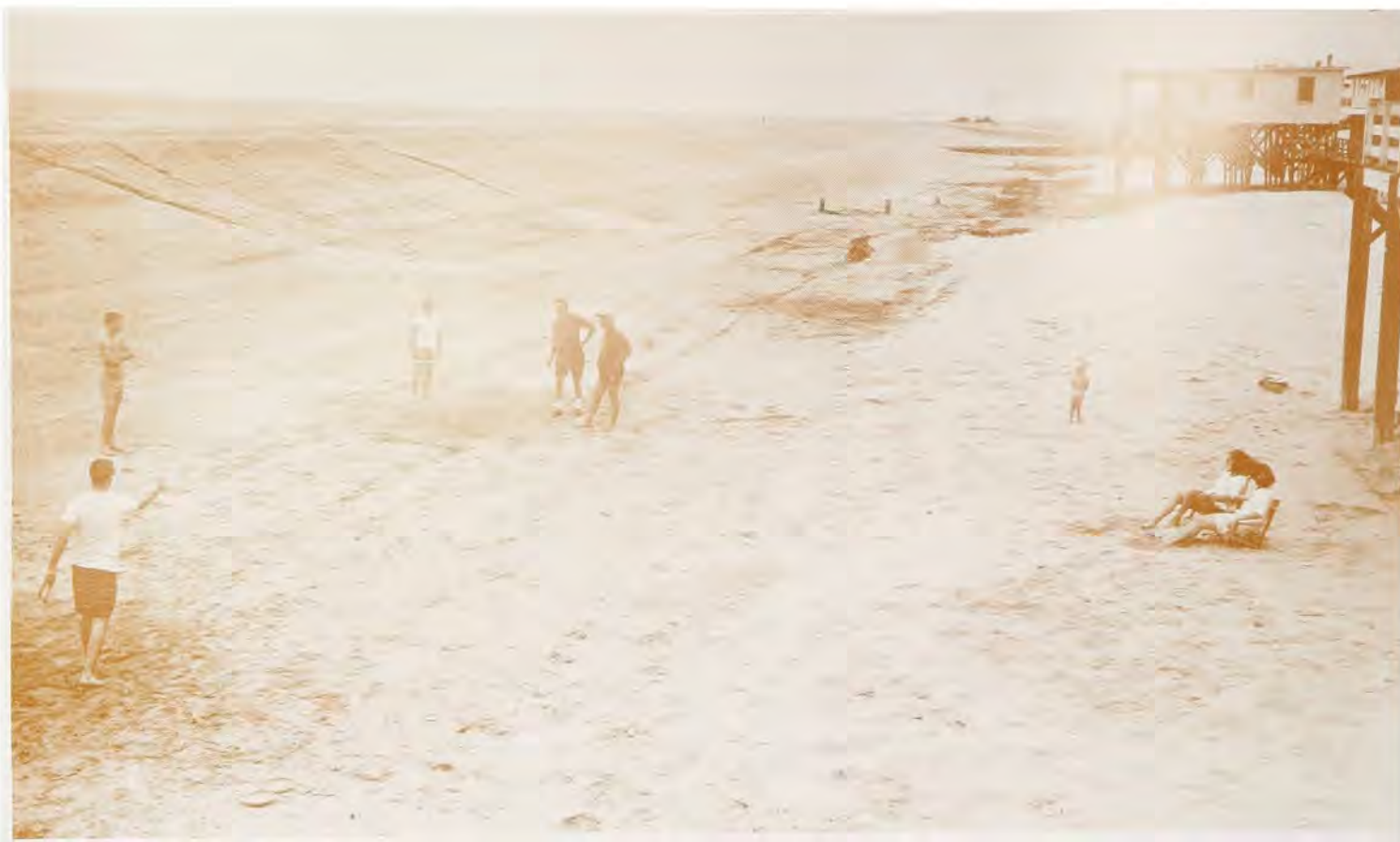
Wrightsville Beach after the berm and dune were constructed, June 1965.
