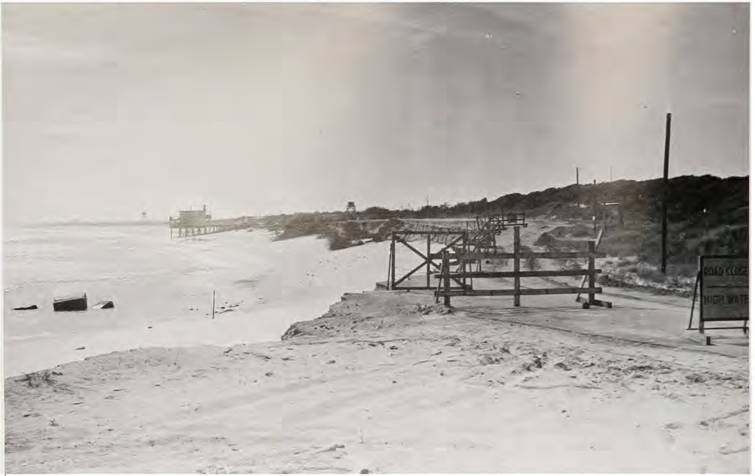
Beach erosion at Fort Fisher looking south, 1946
