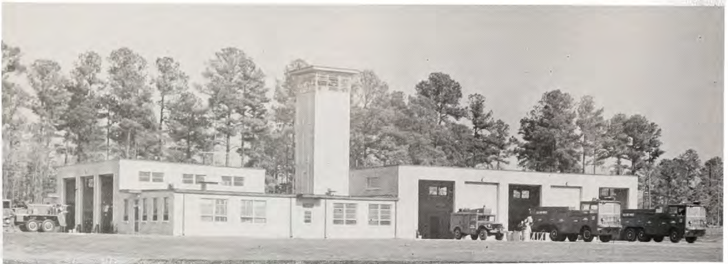
Crash fire station at Seymour Johnson Air Force Base, completed in 1956.
