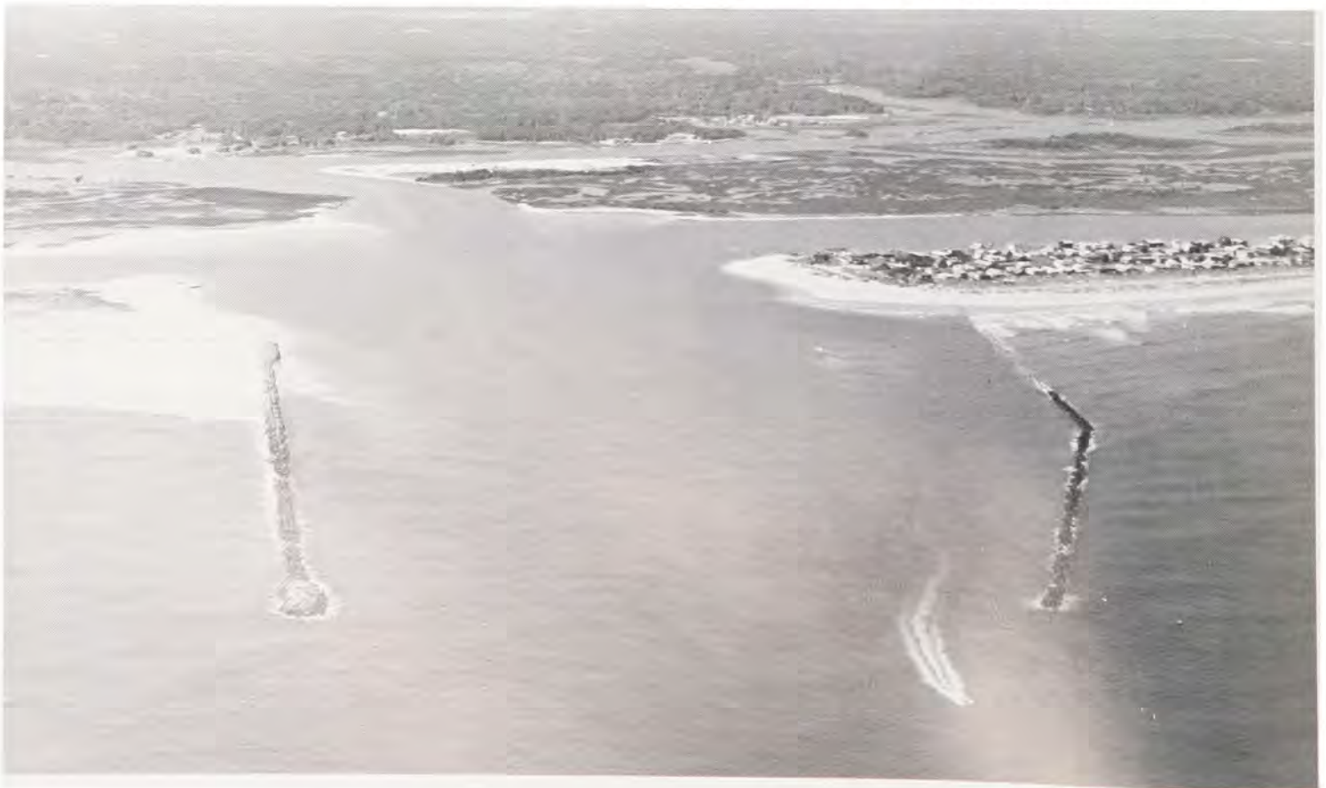
Aerial view of completed Masonboro Inlet jetties
