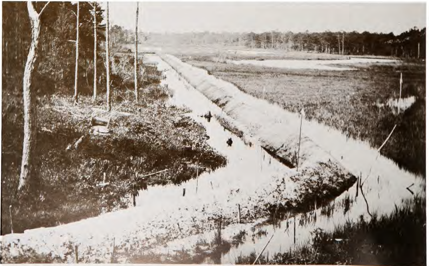
A line was laid out for dredging a portion of the Intracoastal Waterway in North Carolina, 1923.
