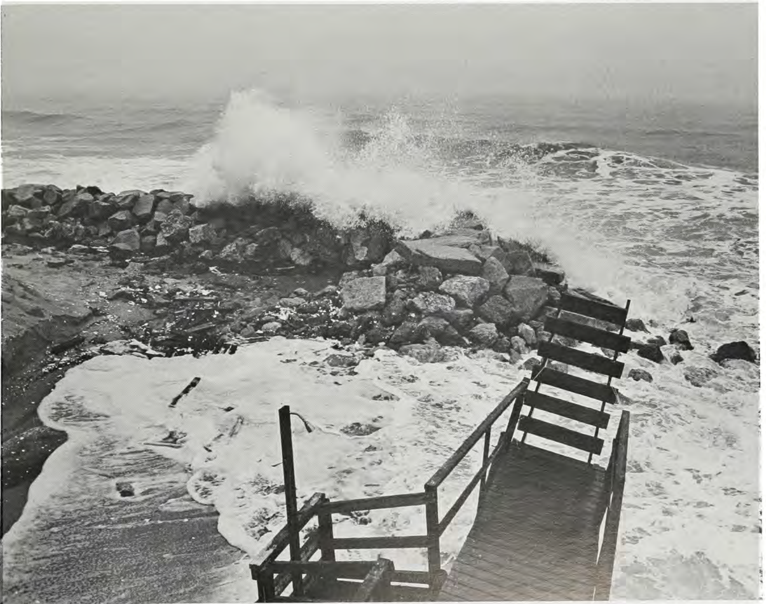
Waves strike Carolina Beach seawall during northeastern storm, December 1980.
