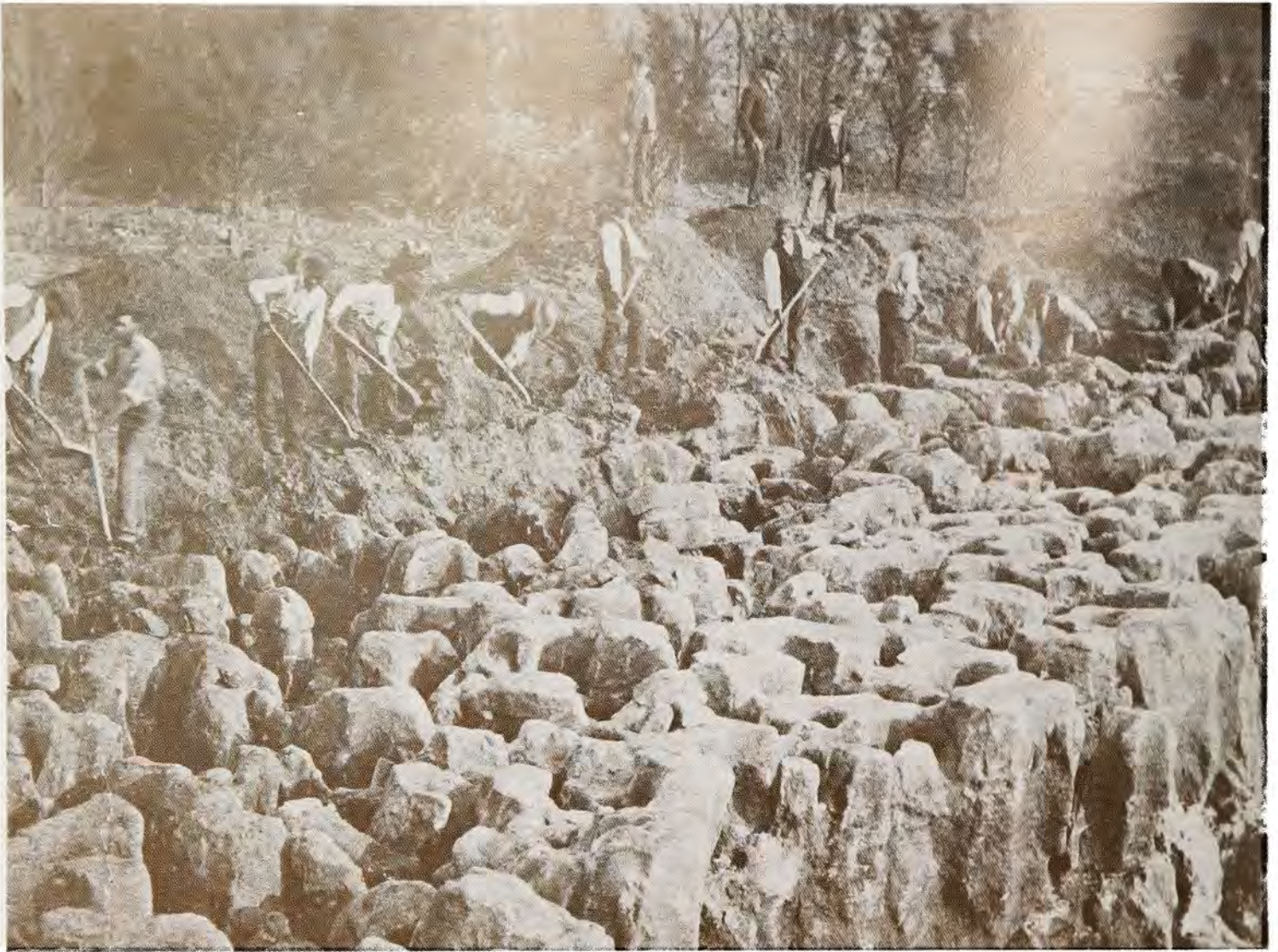
Henry Bacon (upper right), engineer in charge, observed workers using hand tools to uncover stone for use in building the rock dam to close New Inlet. To his right is Colonel Craighill (in civilian clothes) who directed operations in North Carolina from the Baltimore office, c. 1884.
