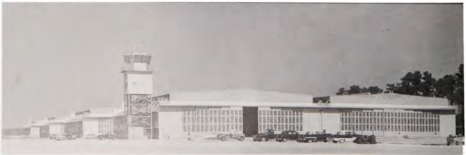
At Seymour Johnson Air Force Base, wooden hangars, constructed during World War II, were restored in 1955.
