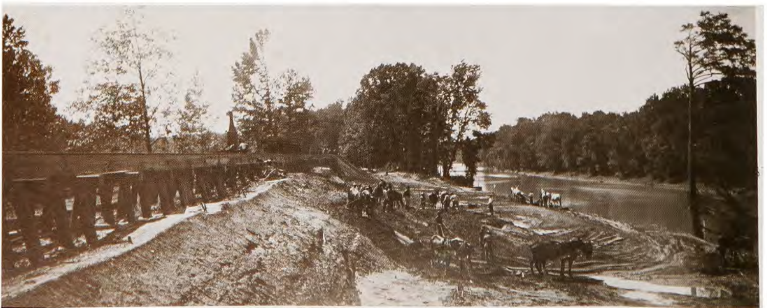
Construction scene at Lock and Dam 2 shows lock site and unloading trestle, 1914.
