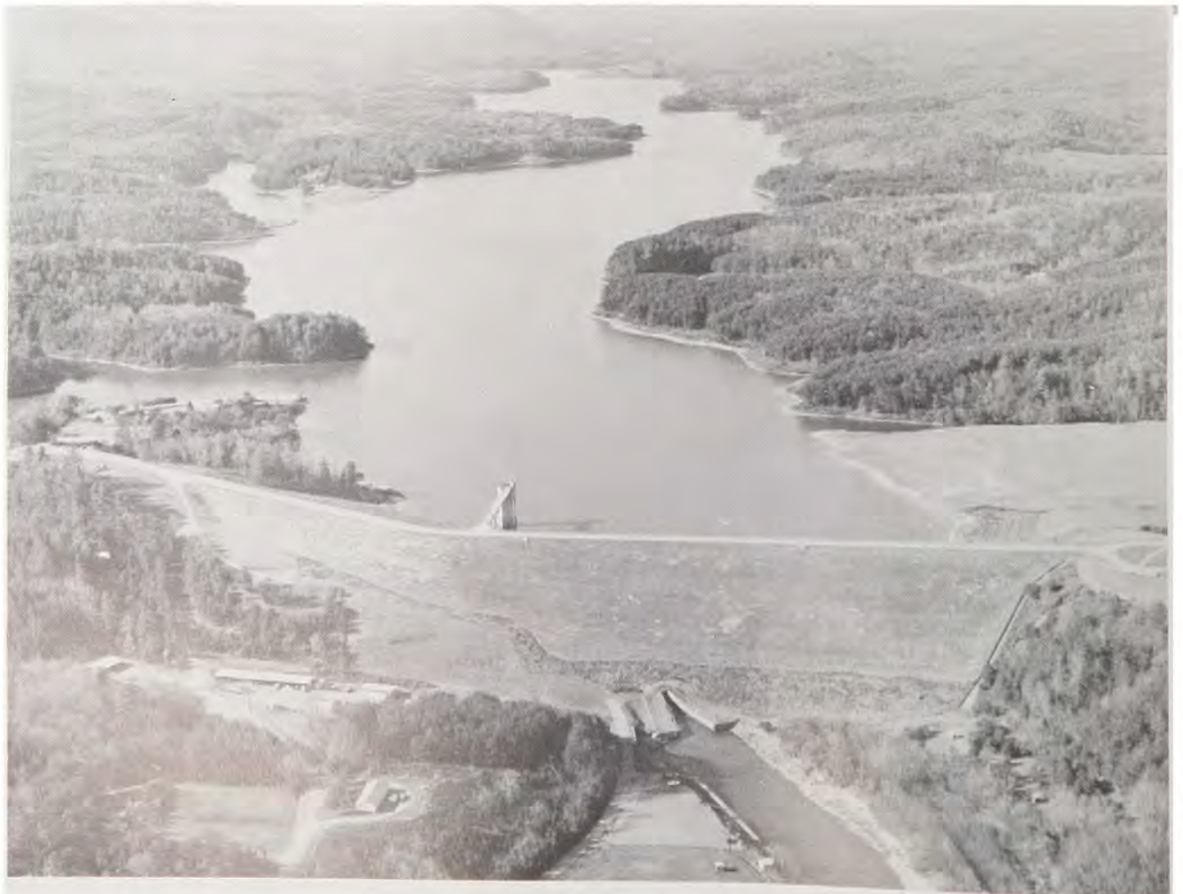
W. Kerr Scott Dam and Reservoir
