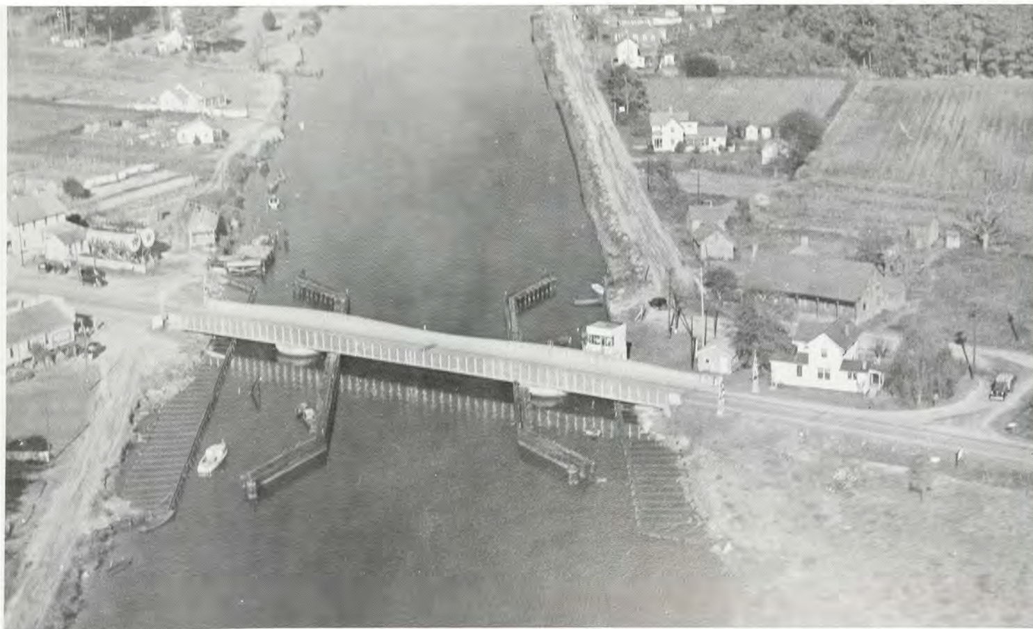
Electrically-operated bridge at Coinjock
