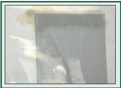
PCMS tile being stripped with CHP
