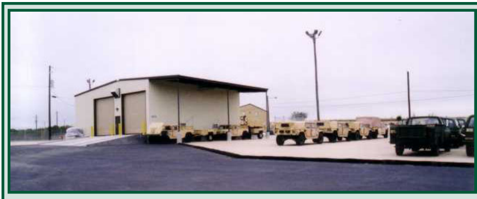
This Corrosion Control Center at Fort Hood will help offset the high corrosion-related operations and sustainment costs associated with fielded vehicles.
