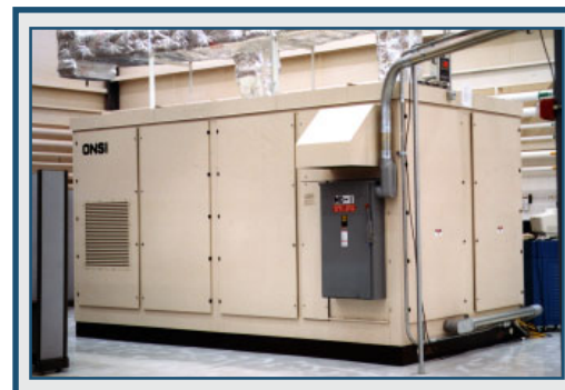
UTC Fuel Cells PC25C, 200 kW Phosphoric Acid Fuel Cell
