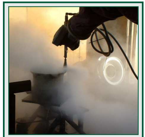
Removal of organic coating using automated UHPWJ
