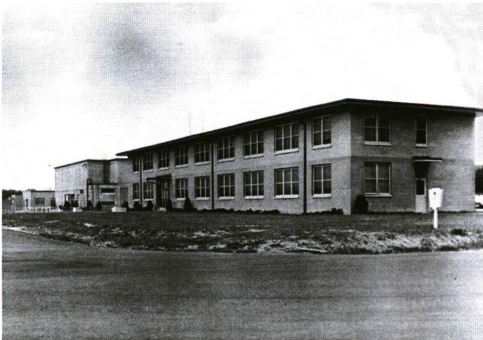
Plate 82: Type 3 Operations Building (foreground) and Modified Type 4 Operations Building (ADCC) (background), 85 th Air Division (Defense), Andrews Air Force Base, 1956. In History of 85 th Joint Air Defense Division and 85 th Air Division (Defense) July – December 1956 , volume 1.
