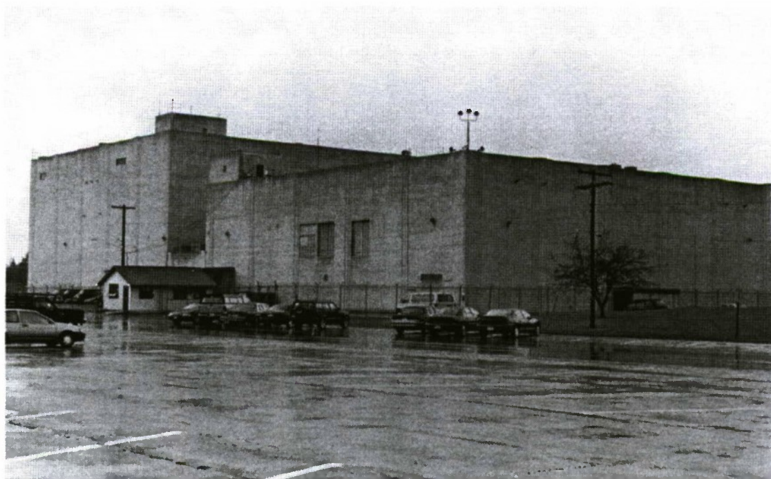
Plate 85: Combat and Direction Centers, SAGE, Syracuse Air Force Station at Hancock Field, 1958. Photograph of July 2000. K.J. Weitze for EDAW, Inc.
