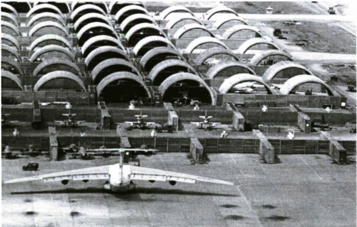
Plate 36: Aircraft Revetments and Concrete Sky Aircraft Shelters, Bien Hoa Air Base, Vietnam. Project Enhance Plus, 9 November 1972. Courtesy of the History Office, Hill Air Force Base.
