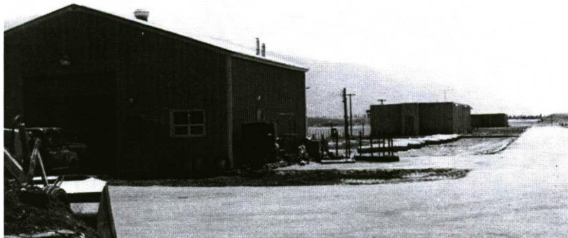
Plate 111: O. Germany. SAC Composite Building and Crew Quarters (Buildings 772, 773, 774, 777, and 778), Satellite Alert, Hill Air Force Base, 1974. In History of the 456 th Bombardment Wing (Heavy) April – June 1974 , volume 1.
