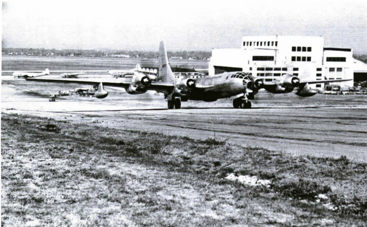
Plate 8: Ten-Percent Inclined Runway, Wright Field, 1942. B-50 on the runway in 1953, with Building 20065 in background. Courtesy of the History Office, 88 th Air Base Wing, Wright-Patterson Air Force Base.
