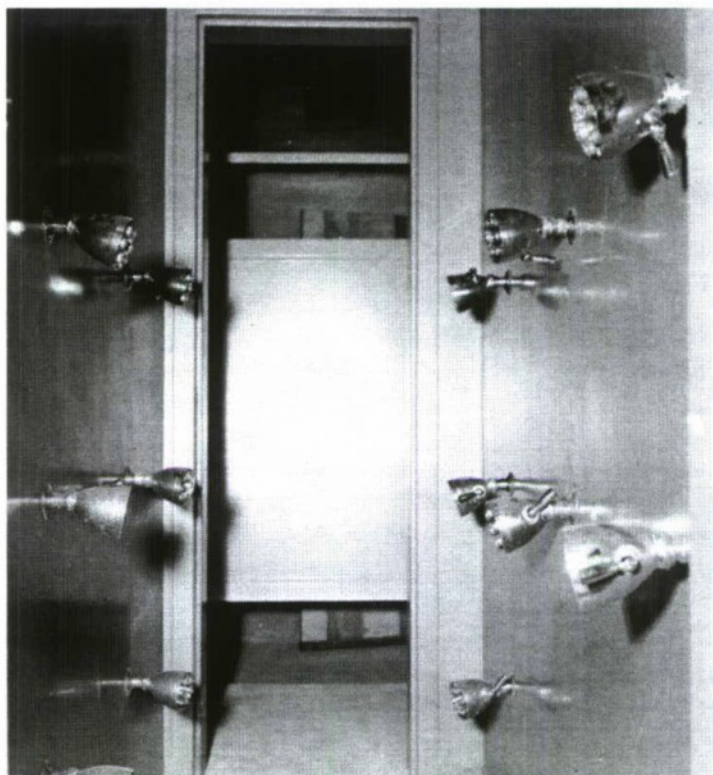
Plate 58: Decontamination Chamber (Showers) in the 27 th Air Division (Defense) ADCC, Norton Air Force Base, 1951. In History of the 27 th Air Division (Defense) 1 January – 31 March 1951 .
