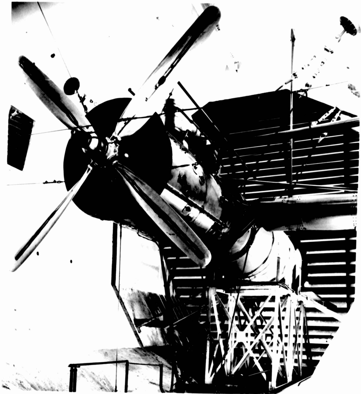
TEST CELL INSTALLATION PRATT & WHITNEY XR-4360-A ENGINE
