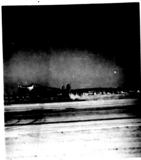
Fig. 45 -- Biplane assisted by auxiliary jet propulsion at start of climb after take-off.
