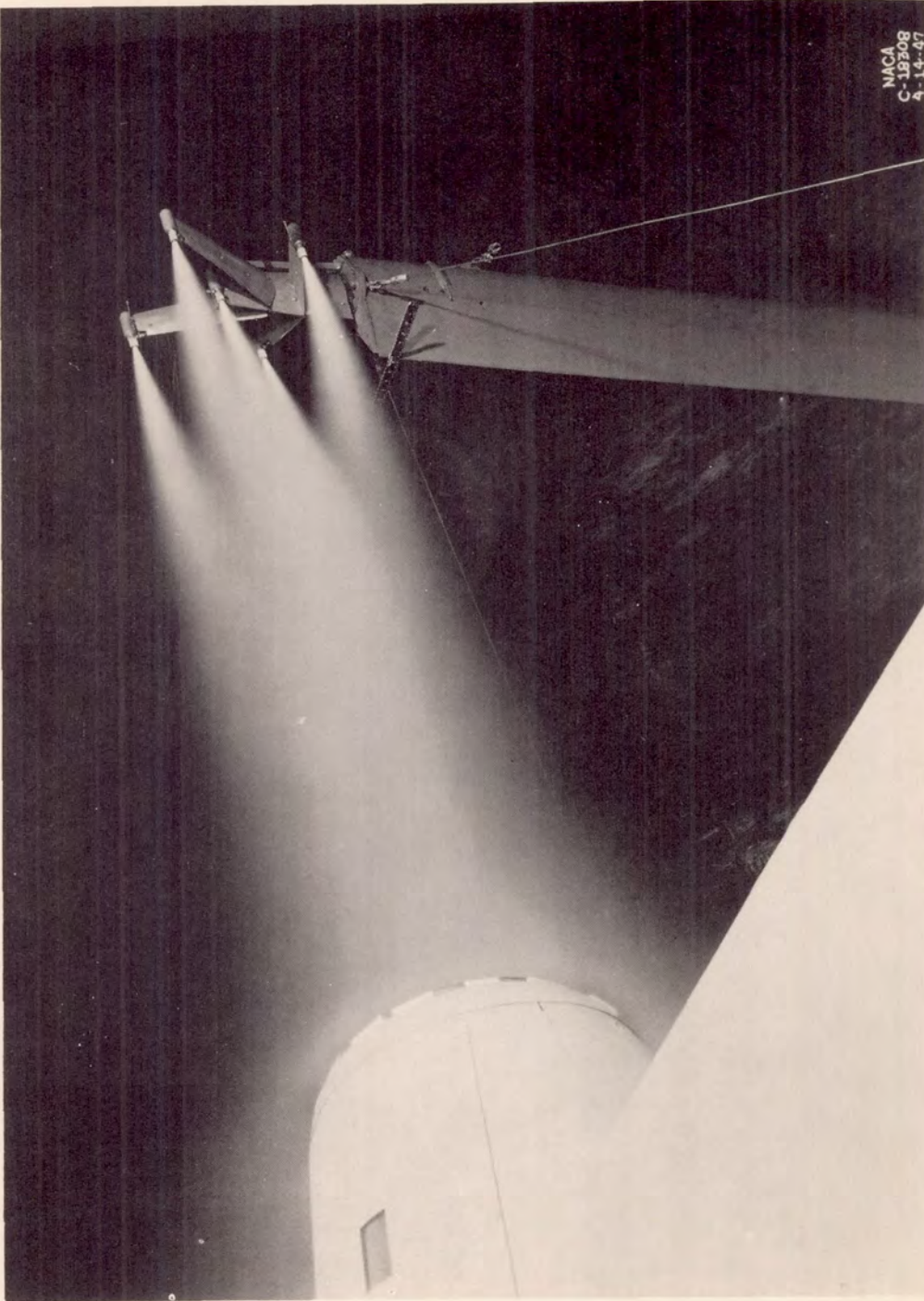
INLET ICING SPRAY FIGURE 3.
