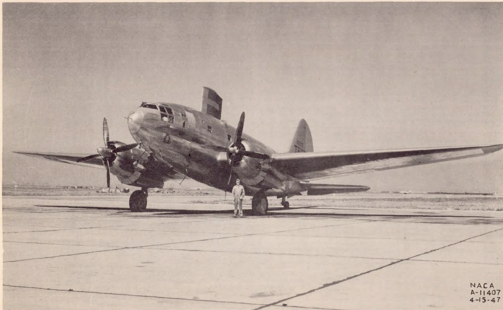
Figure 1.- The C-46 airplane as equipped for icing flight research and operated by the Ames Aeronautical Laboratory during the winter of 1946-47.
