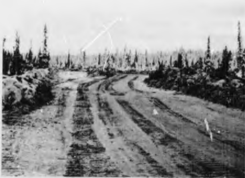
Figure 14 (Part V) to Section IV. Finished road, compare to Figure 9.
