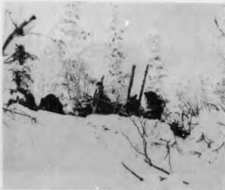
Figure 12 (Part V) to Section IV. Loose Timber used as Parapet.
