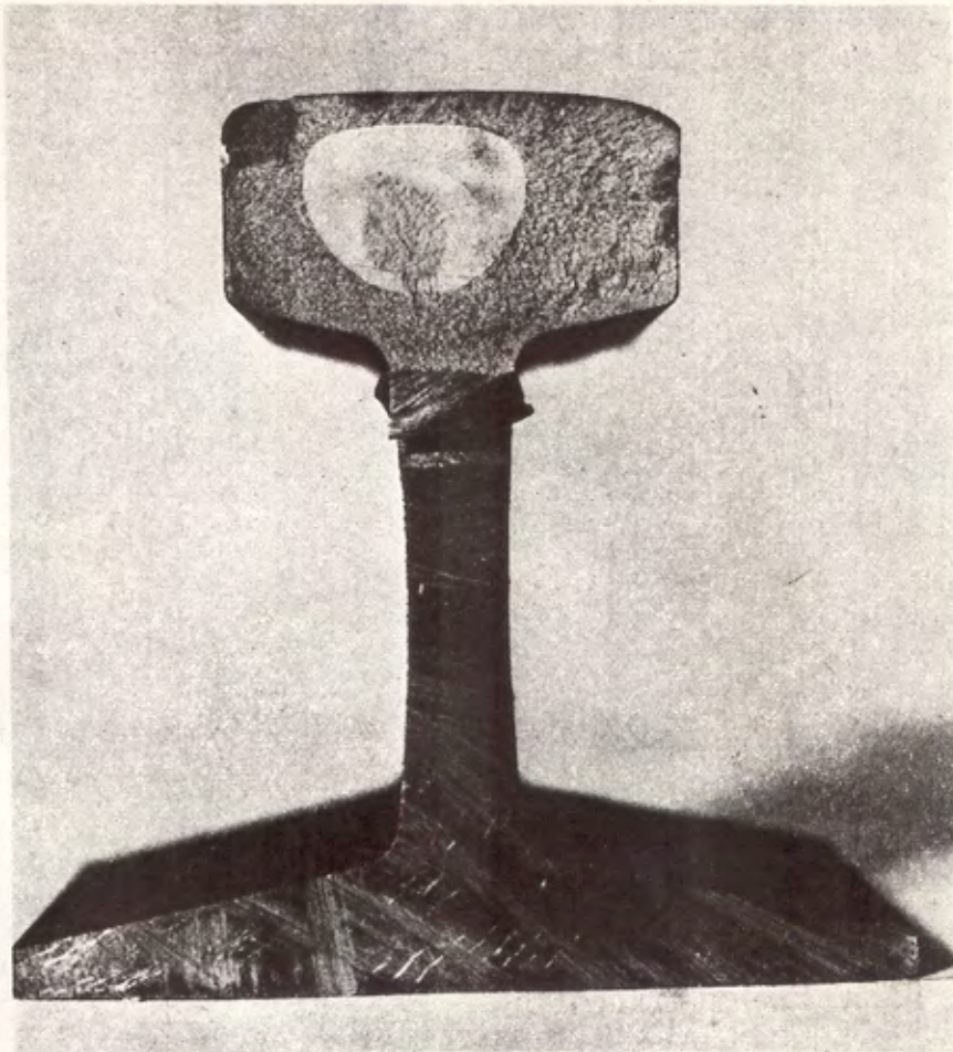
FIG. 33.—Transverse Fracture in Rail. (Courtesy Sperry Rail Service, Sperry Products Corp., Danbury, Conn.)
