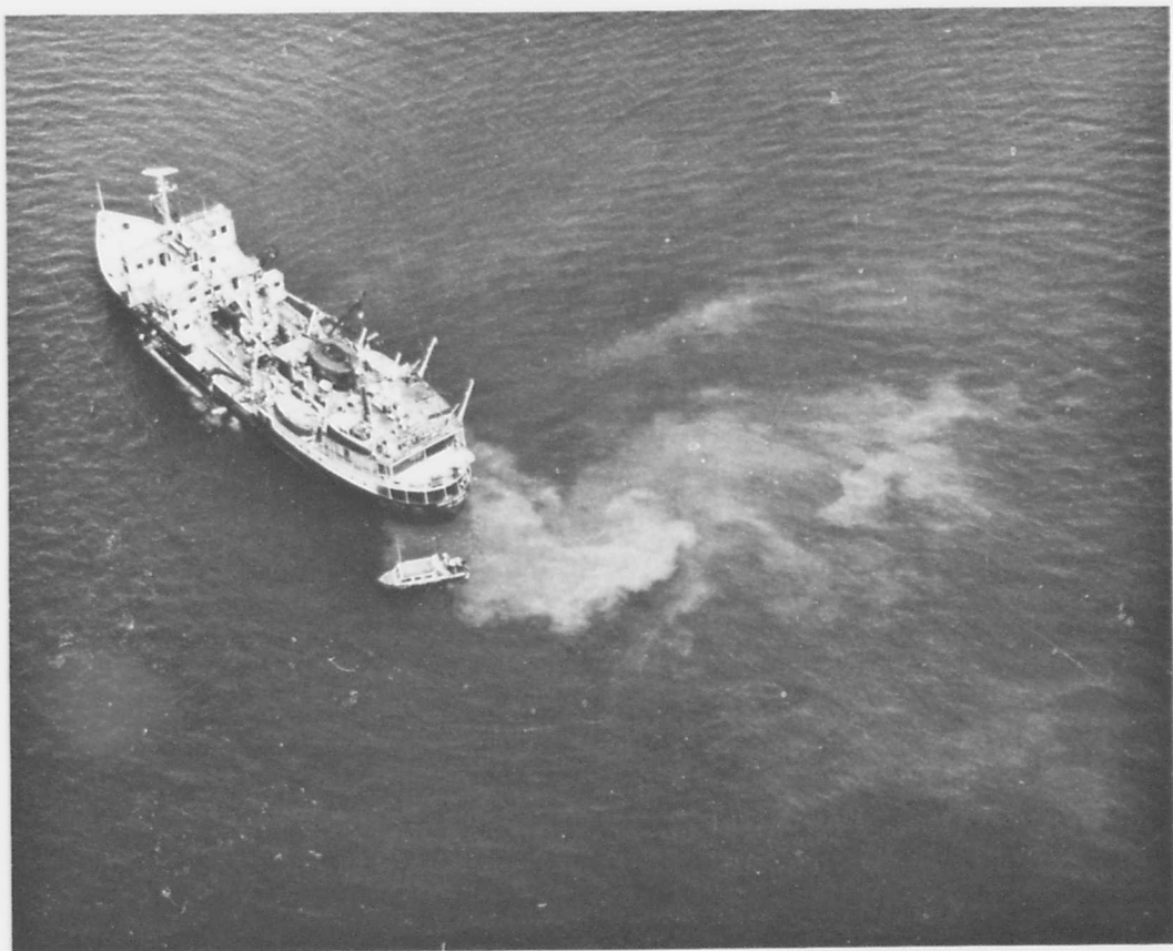
Photo 22 Stationary Open Lake Disposal by Hopper Dredge
