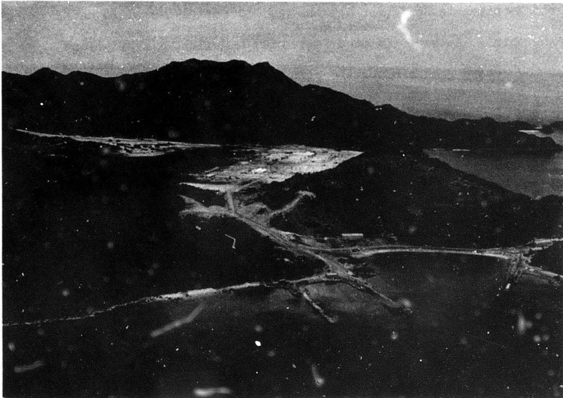
The piers and base at Cam Ranh Bay.
