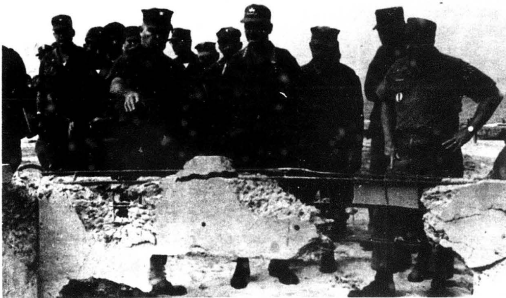
Rear Admiral J. V. BARTLETT, Commander, Third Naval Construction Brigade, points out the results of destructive tests held on sections of precast concrete bunkers to General W. C. WESTMORELAND (center), Commander, U. S. Military Assistance Command, Vietnam, and Lieutenant General R. E. CUSHMAN (right), Commanding General, Third Marine Amphibious Force.
