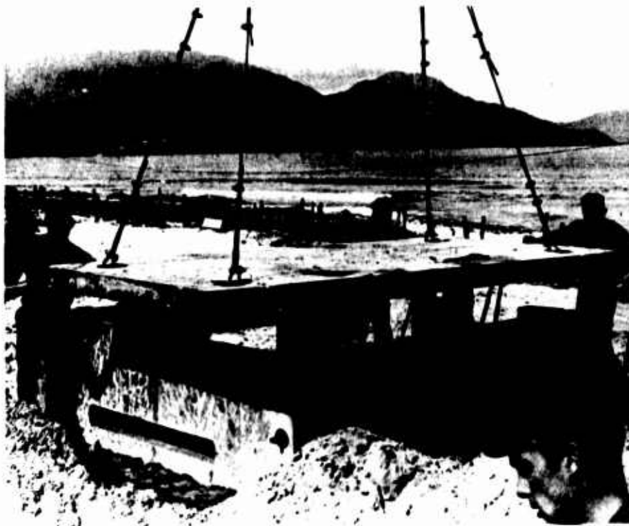
Seabees from MCB 1 erect a precast concrete bunker near the THIRD Naval Construction Brigade Headquarters at Red Beach.
