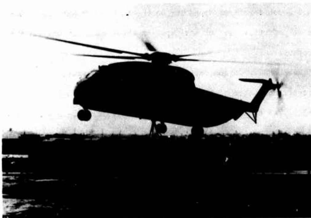
A Marine CH-53 helicopter hooks up to a Seabee "dozer" for a rapid transport to a remote construction site in northern Quang Tri province.
