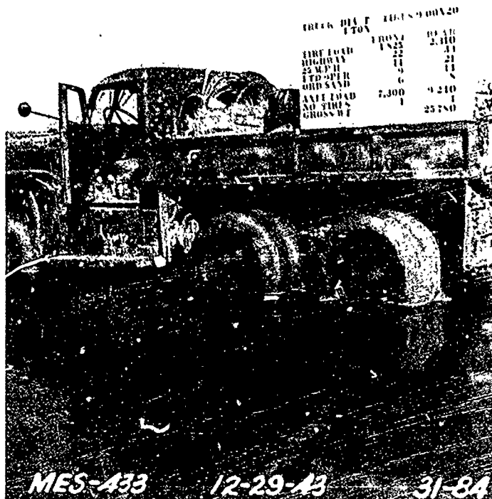
TIRE TESTS IN MUD. Four ton Cargo truck with 9.00-20 tires at Ordnance Sand Min- imum Inflation stuck in the mud. Note the depth of water in this area.
