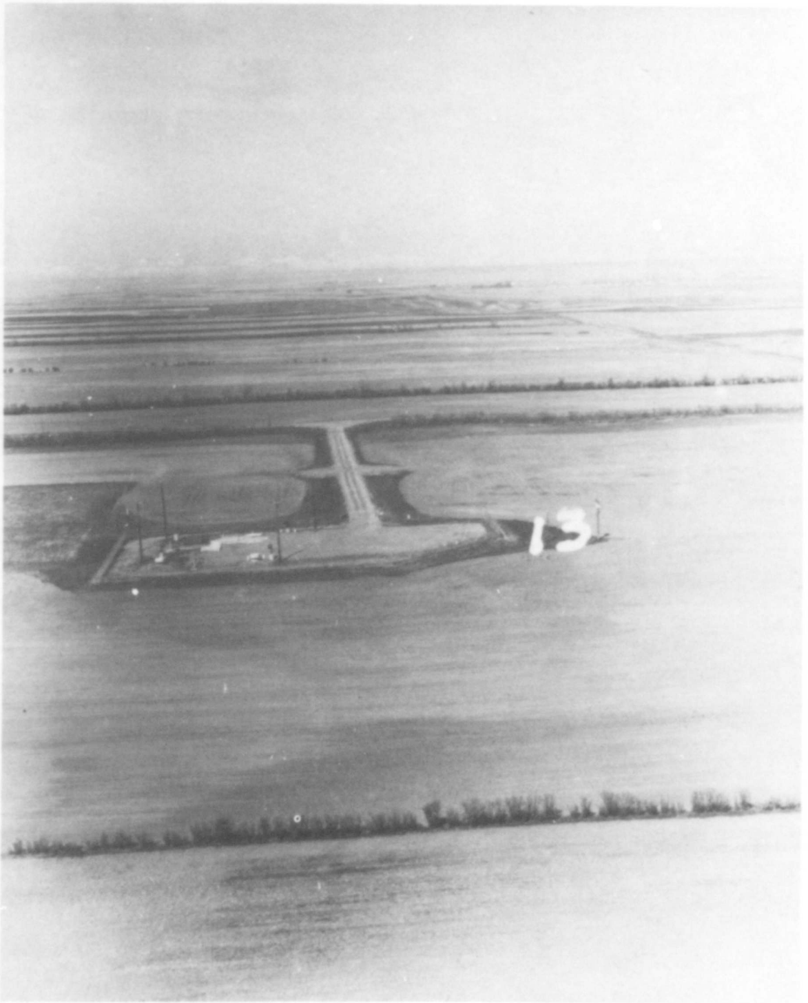
Figure 2-3. LAUNCH FACILITY SIERRA 40 LOOKING WEST
