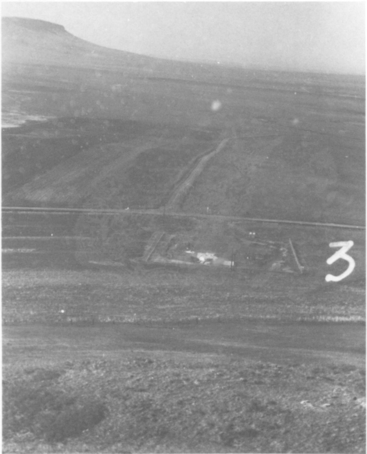
Figure 2-4. LAUNCH FACILITY GOLF 3 LOOKING WEST
