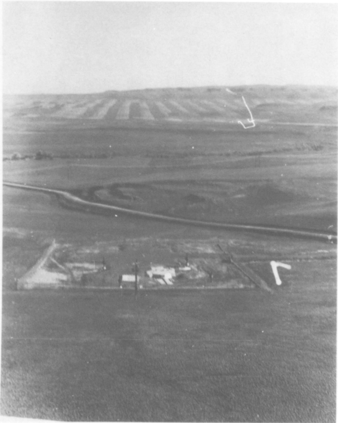
Figure 2-5. LAUNCH FACILITY GOLF 4 LOOKING WEST
