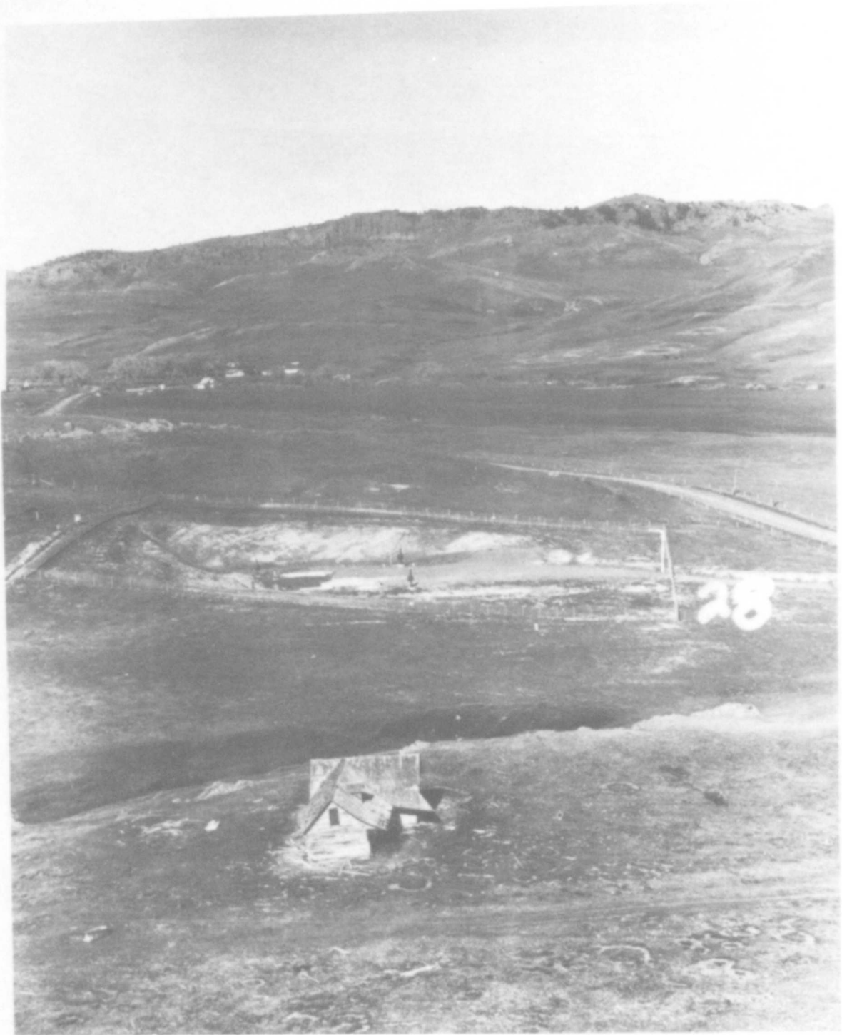
Figure 2-6. LAUNCH FACILITY GOLF 5 LOOKING WEST
