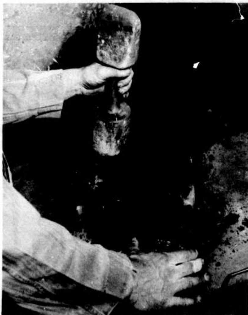
Figure 103. Ramming up the core.
