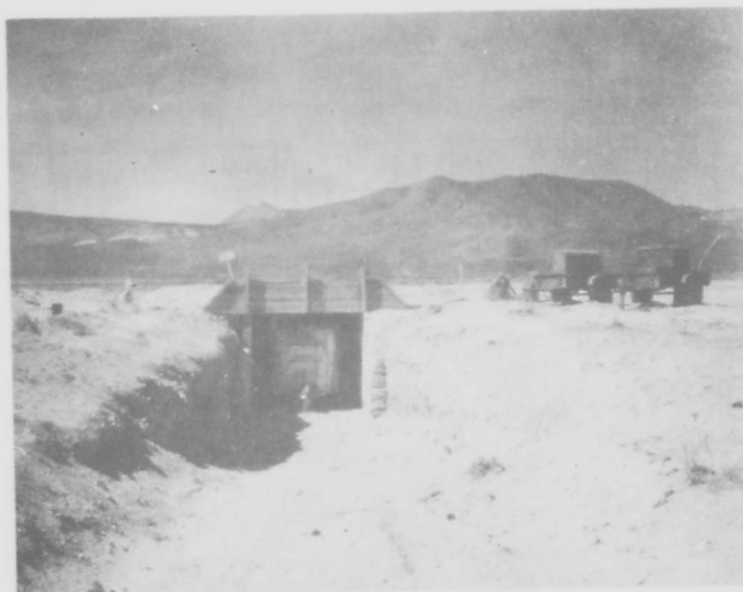
Fig. 3.8 Recording Trailer in Shelter. Portable generators shown at right
