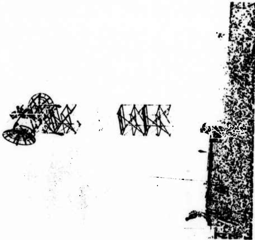
(7) Figure 24 Mounted parabolic reflectors, used for microwave link.
