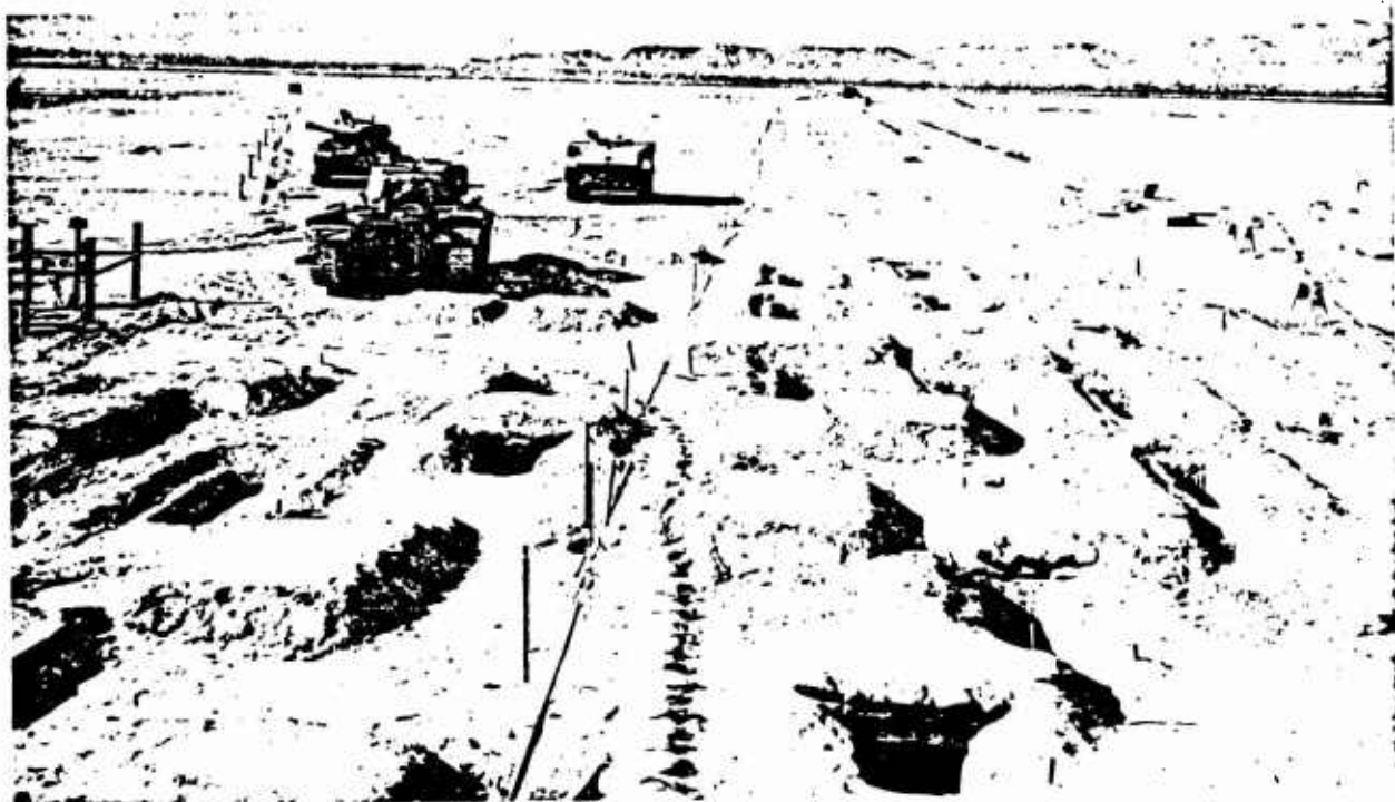
Figure 2.6 North axis array, Subproject 4.2.1.
