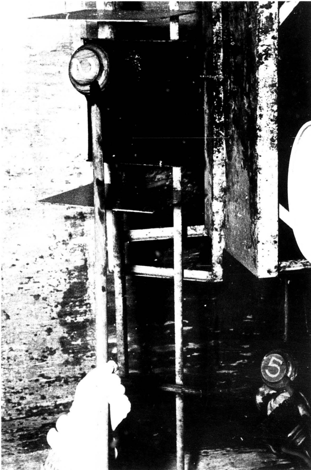
FIG. 2.14 Brushing Technique Used in Investigation of Industrial Decontamination Procedures
