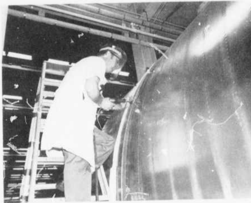
FIGURE 140 — CENTER SECTION OF FUSELAGE SIDE PANEL BEING REMOVED
