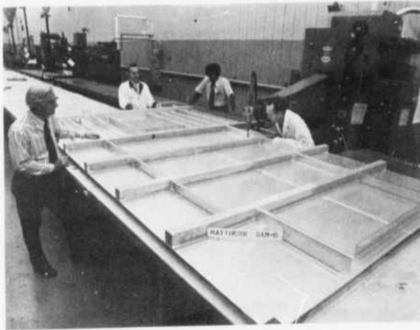
FIGURE 105 — TACK WELDING A SIDE SECTION OF THE RAYTHEON SHELTER PRIOR TO ROLL SPOT WELDBONDING
