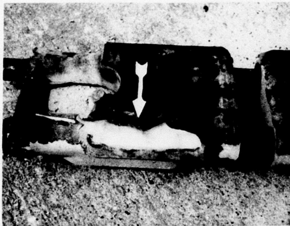
Figure 4. Arrow Denotes Pin Tube Wear Due to Failure of Road Wheel Path Rubber
