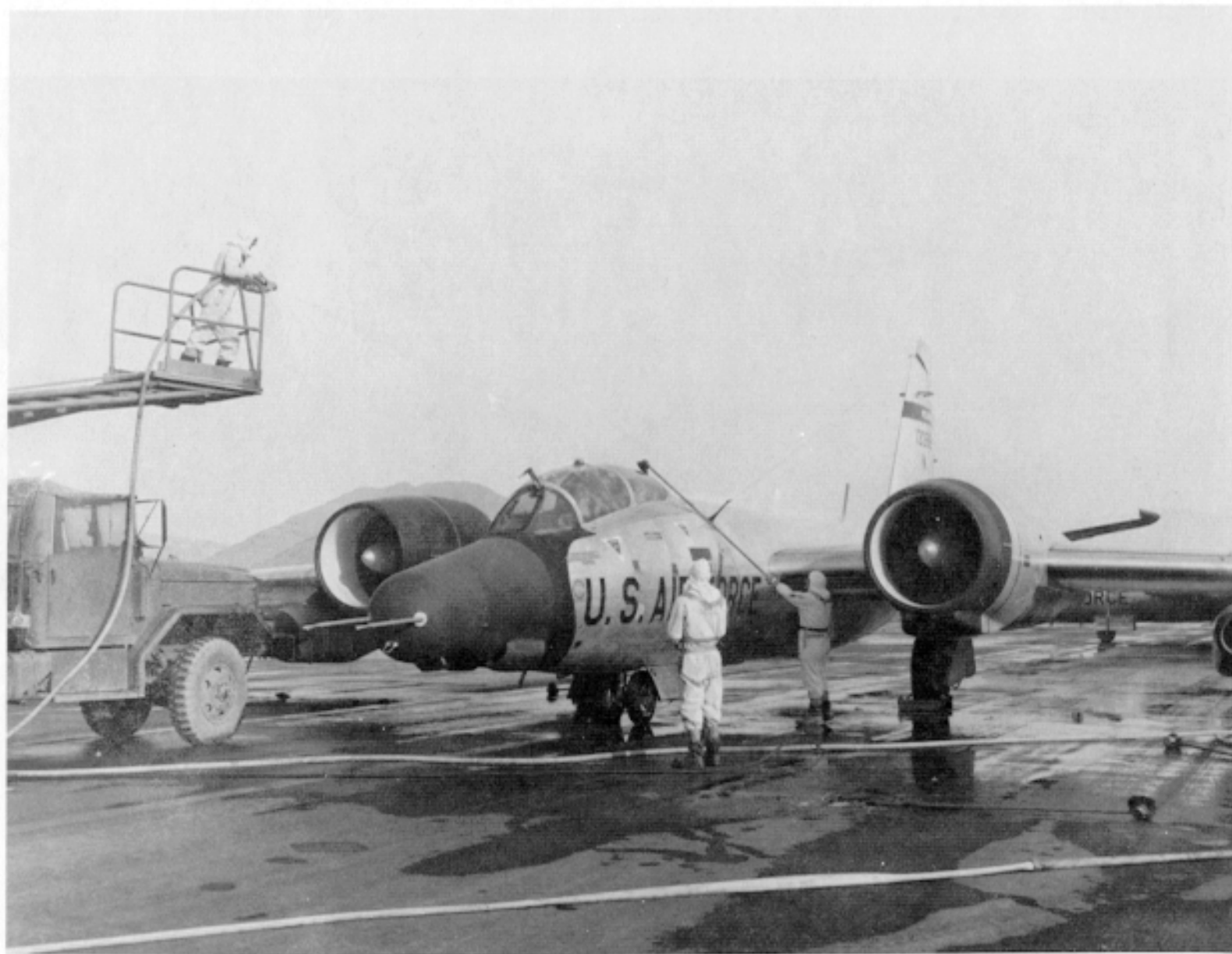
Figure 2.7 Air Force personnel decontaminating a B-57 cloud sampling aircraft.
