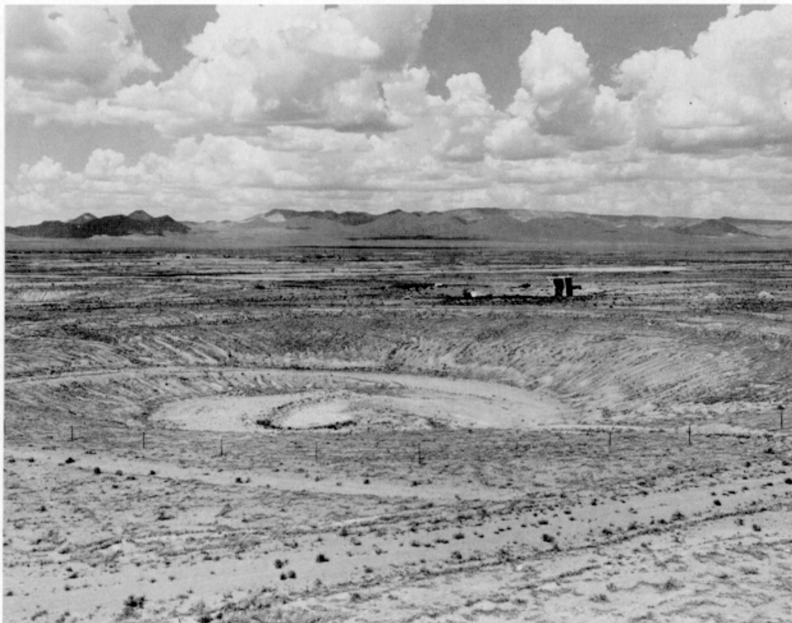
Figure 2.1 A typical subsidence crater.
