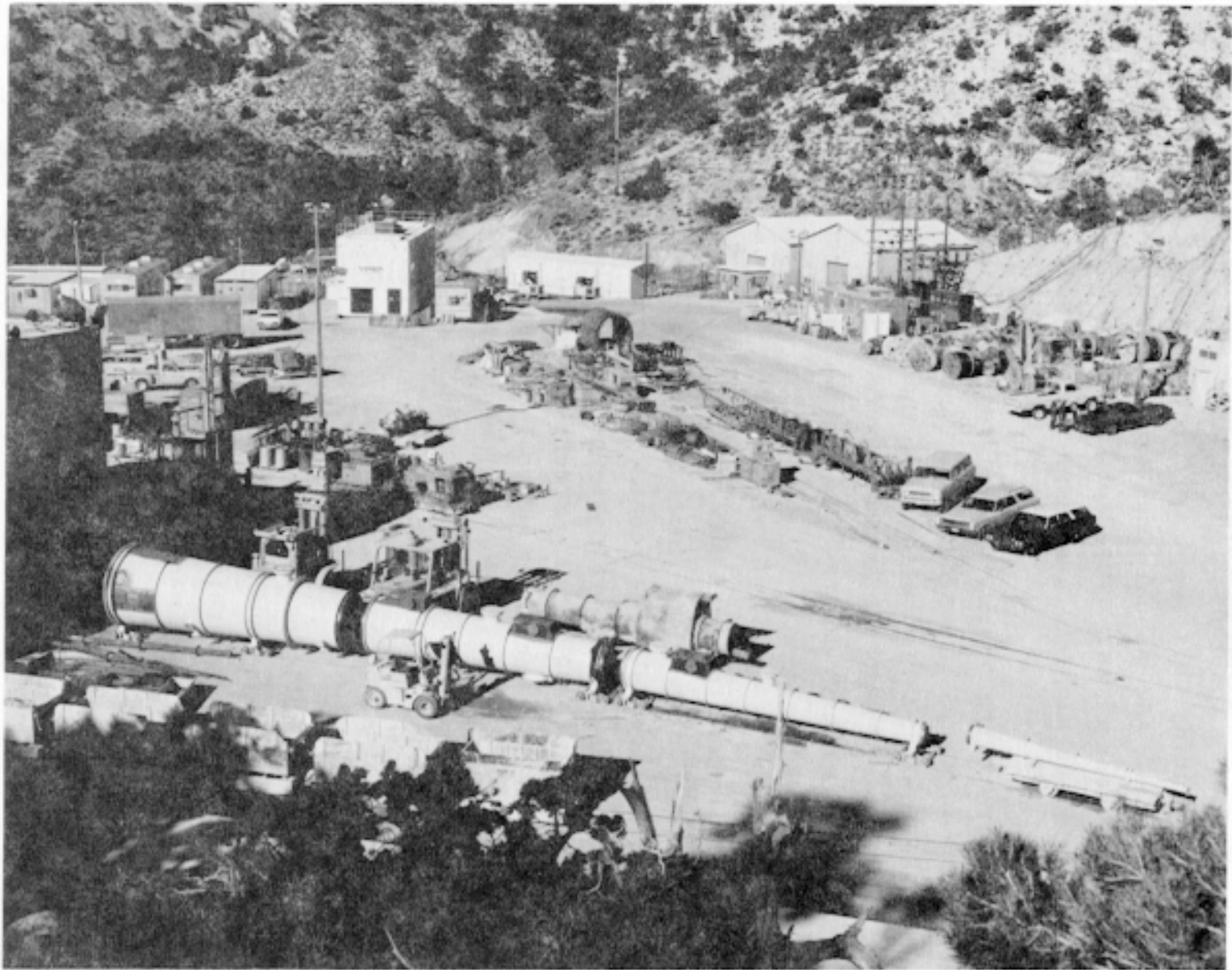
Figure 7.3 HYBLA FAIR Event - HLOS Pipe Sections
