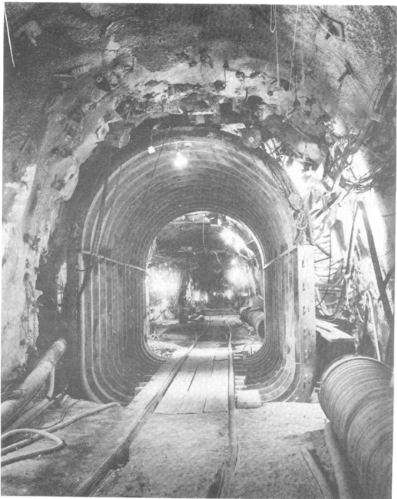
Figure 8.2 MINERS IRON event - OBP before concrete pour.
