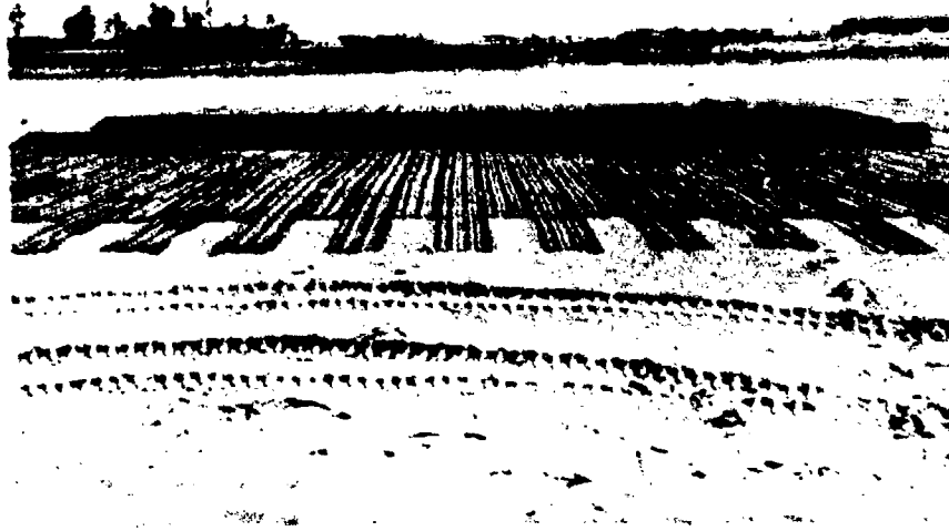
C. Side top view of pit showing landing mat next to sides of pit to support the main landing gear wheels of the B-29 airplane.
