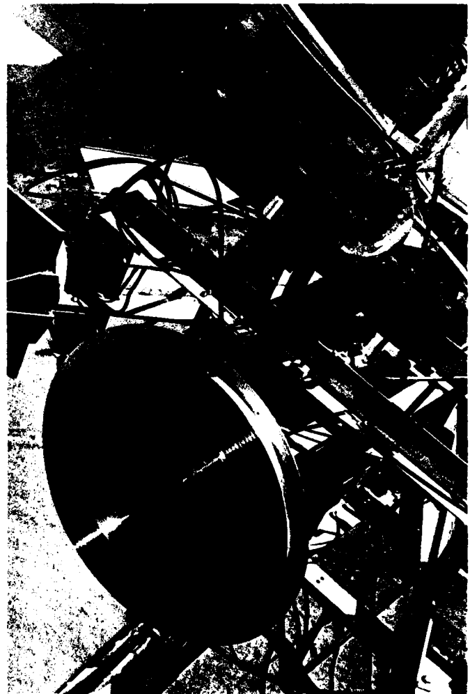
Figure 26. Shaped beam feed installation
