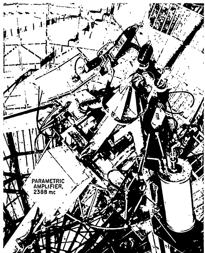
Figure 86. Parametric amplifier installed at feed-point
