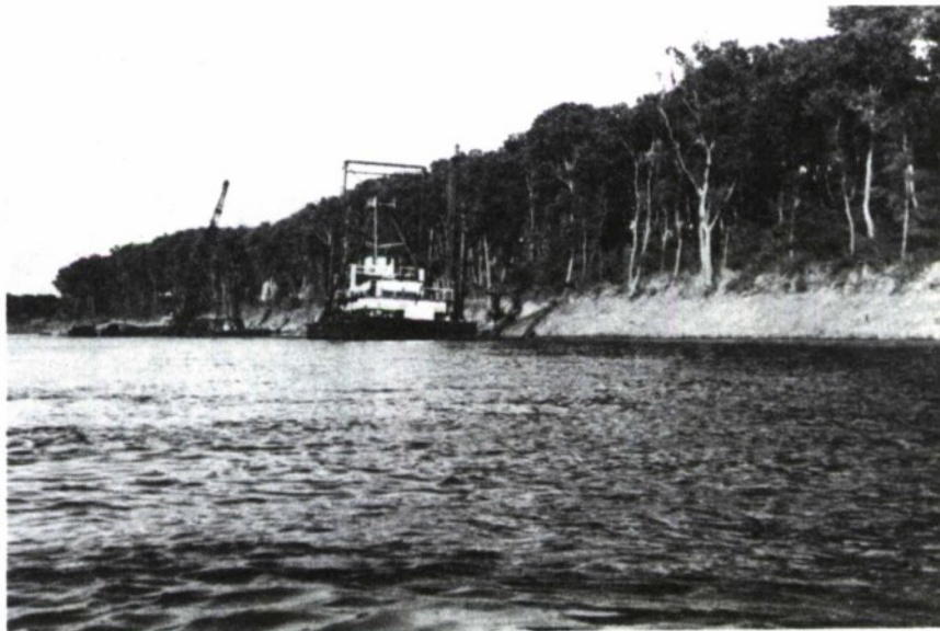
Figure 9. Waterside placement of stone revetment allows retention of riparian vegetation on levee berms.
