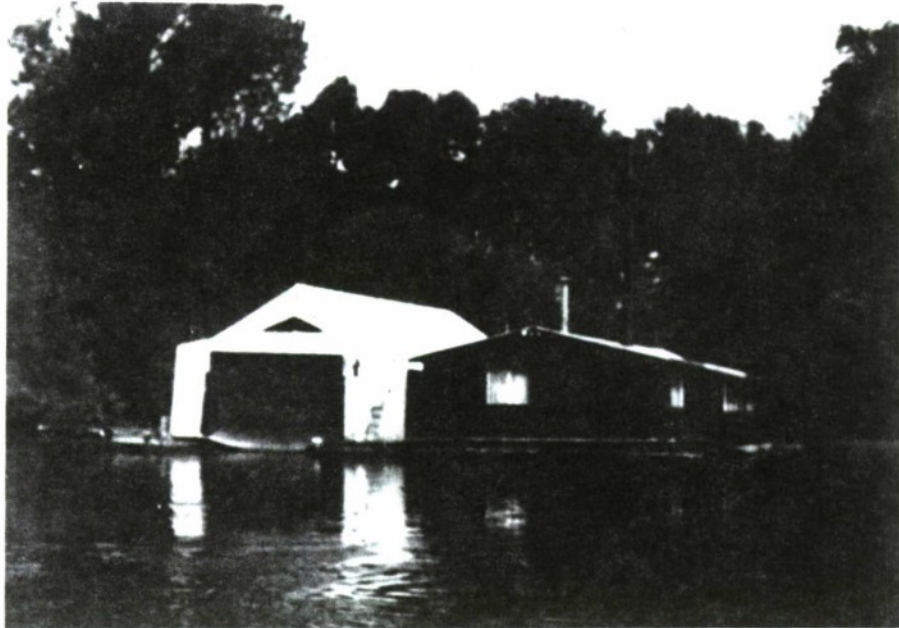
Figure 13. Floating houses and boat docks not only intrude upon the river and seriously degrade the environmental integrity, but they preclude the use of the area by the public at large for fish and wildlife resources.
