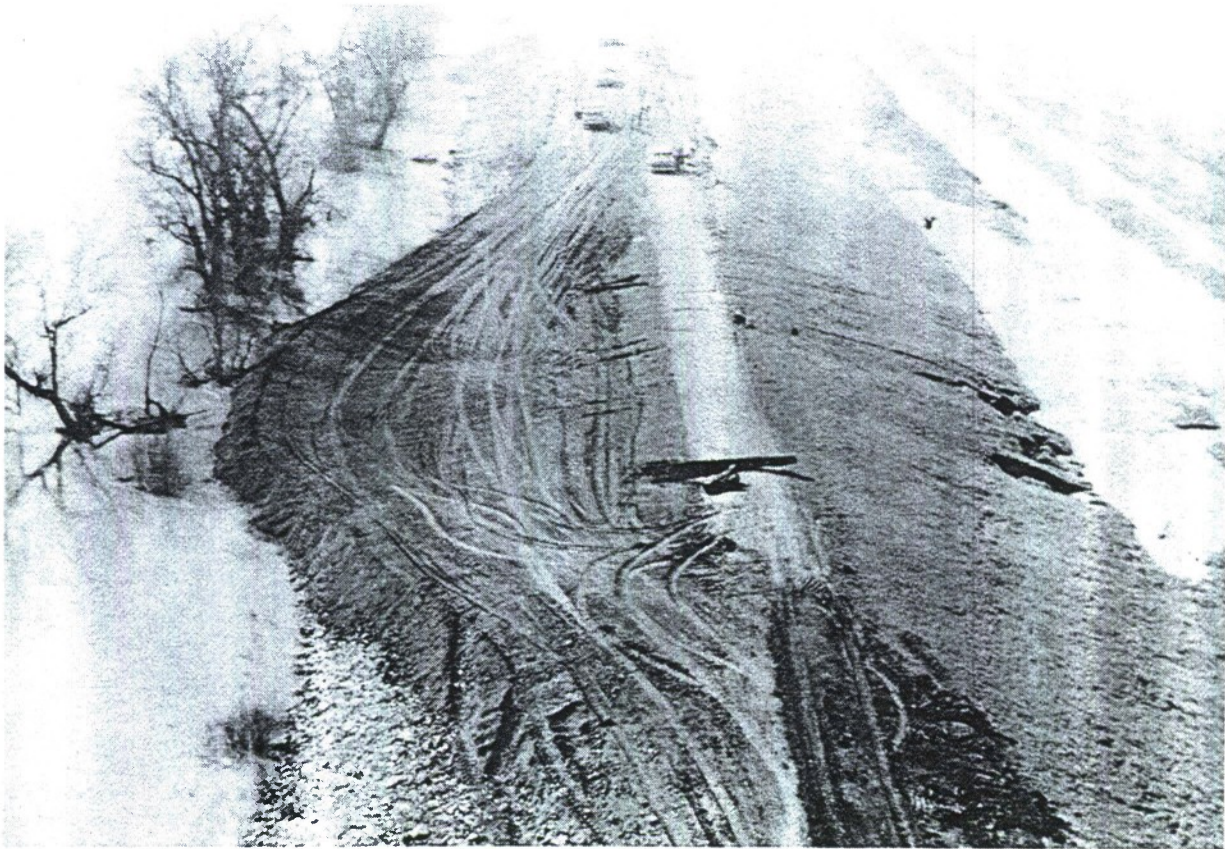
EMERGENCY FLOOD FIGHT EFFORTS ON WEST LEVEE SUTTER BYPASS DURING FEBRUARY 1986 FLOOD.
