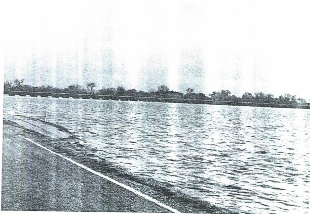
FEBRUARY 1986 FLOODFLOWS EXCEEDED DESIGN CONDITIONS FOR SACRAMENTO WEIR AND BYPASS.
