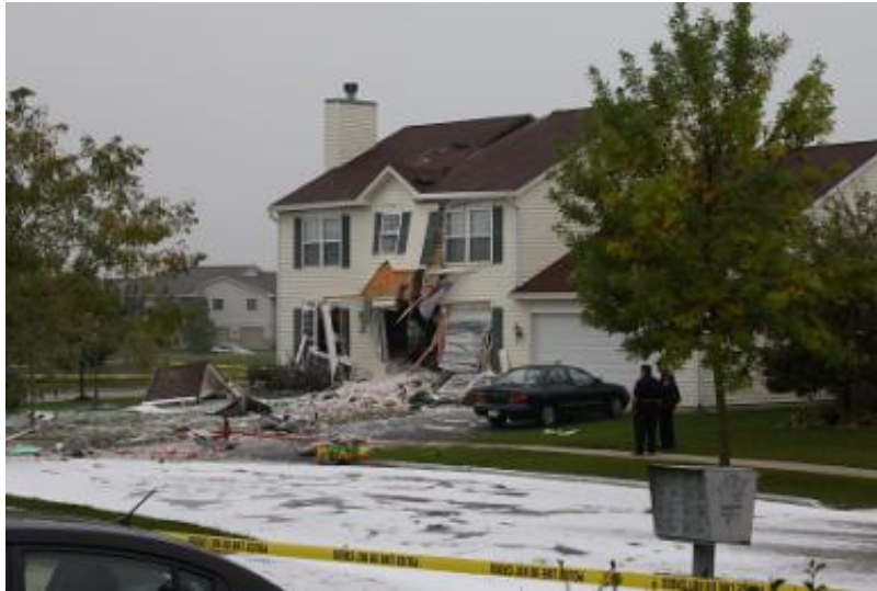
Figure 35: Residential House Impacted by Helicopter
