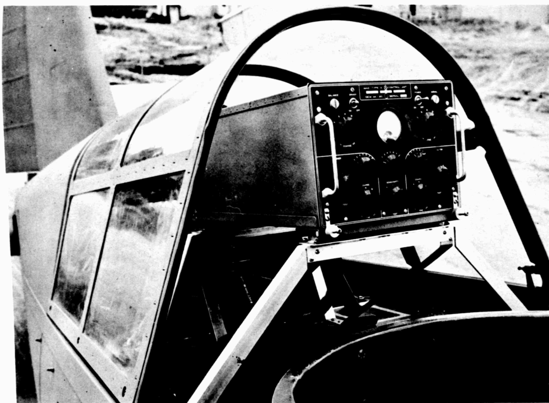
AM-1/ASQ-1 INSTALLED BEHIND OBSERVER'S SEAT IN AN OS2U AIRPLANE FIGURE 32
