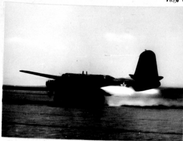
Fig. 29 -- Assisted take-off during ground run. Side view showing size of jet blast.
